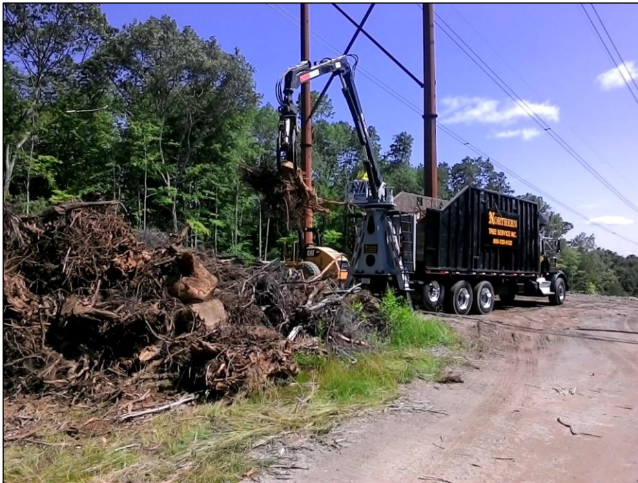
Photo #7: Stump removal at Str 199 as part of restoration operations. (7/16)
