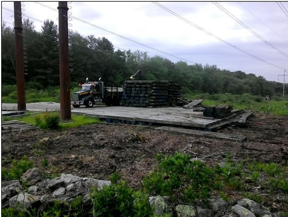
Photo #4: Mat removal at Str 153. (7/9)
