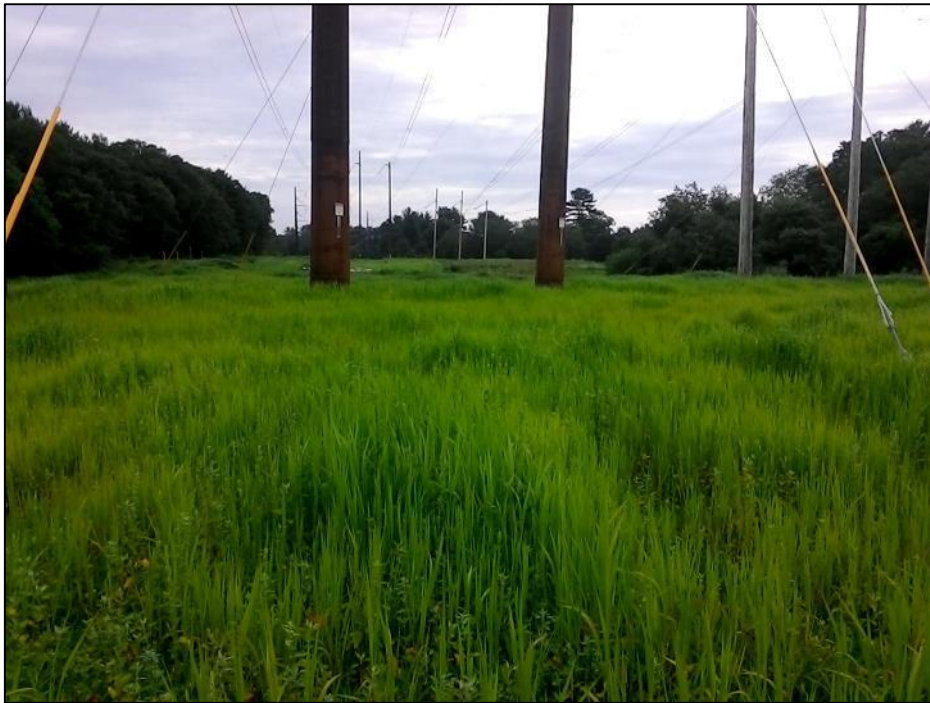
Photo #1: Str 78 fully stabilized. (7/9)
