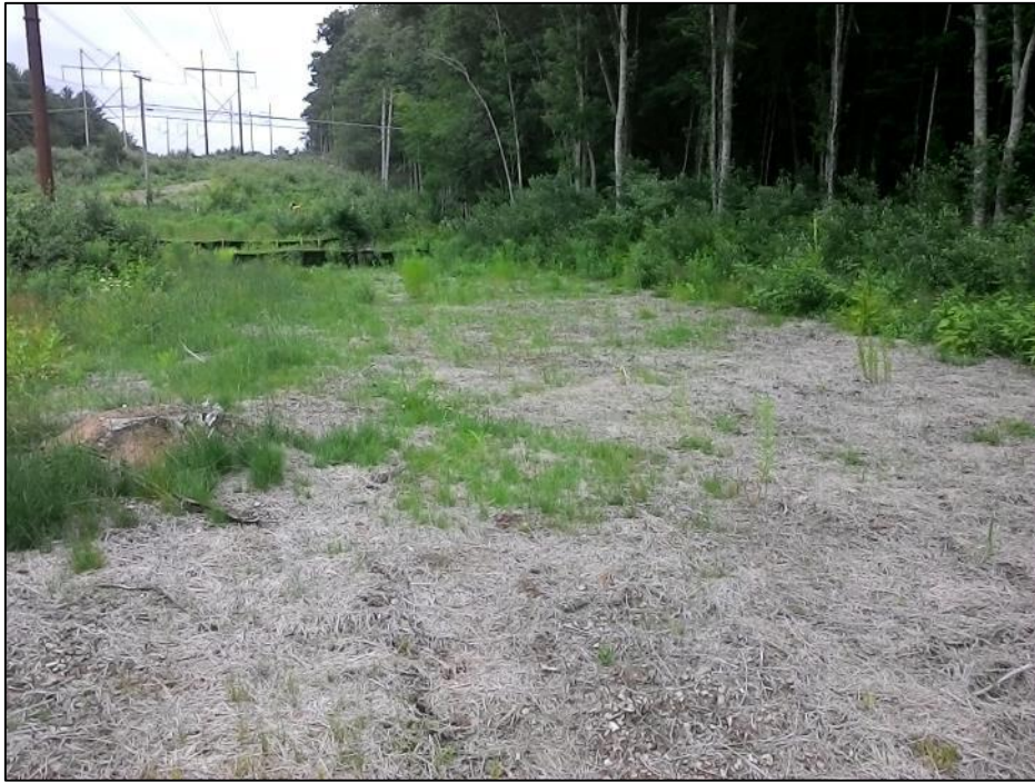
Photo #3: Str 91 not yet stabilized. (7/9)
