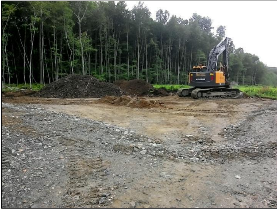
Photo #5: Restoration Operations at Str 159. (7/9)
