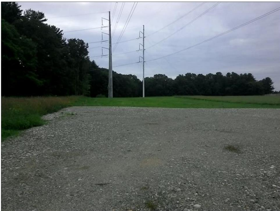
Photo #2: Str 83 not yet stabilized. (7/9)
