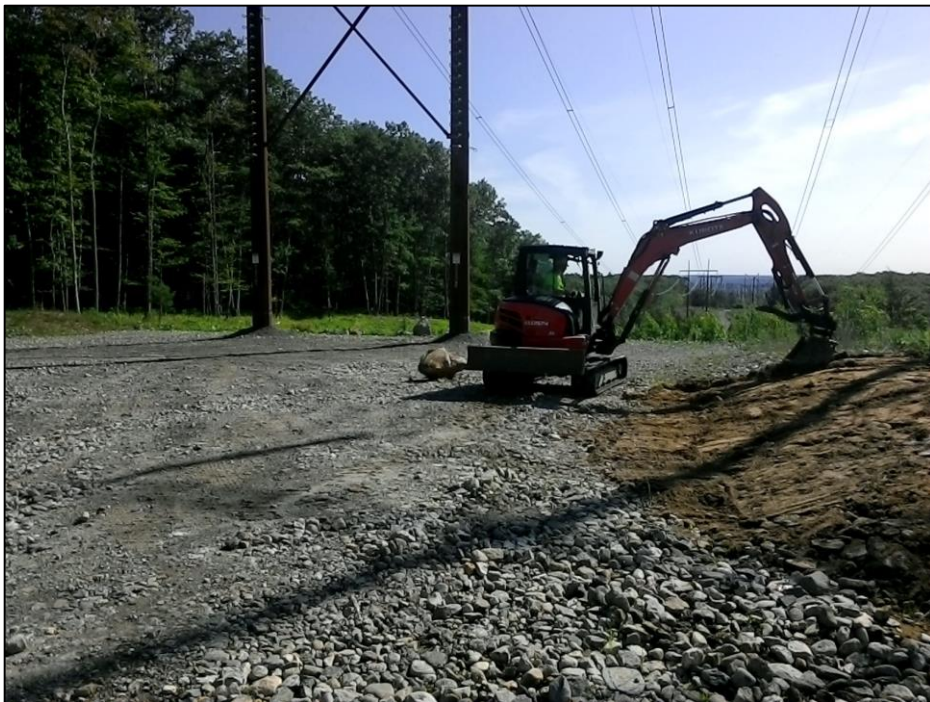
Photo #6: Restoration operations at Str 171. (7/16)
