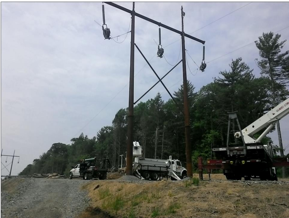
Photo #2: Stringing operations at Str 309. (6/11)
