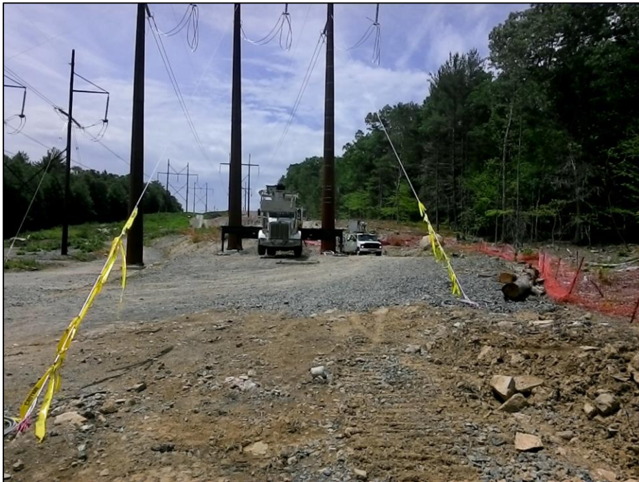
Photo #8: Preparing fiber optics at Str 337. (6/18)
