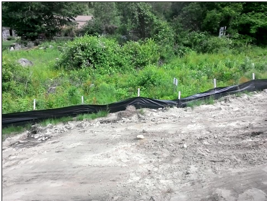
Photo #10: Silt fence re-stapled. (6/18)
