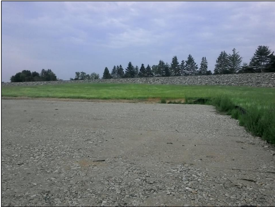
Photo #3: Geotextile fabric and other debris on pad between Str 82 and 83. (6/11)
