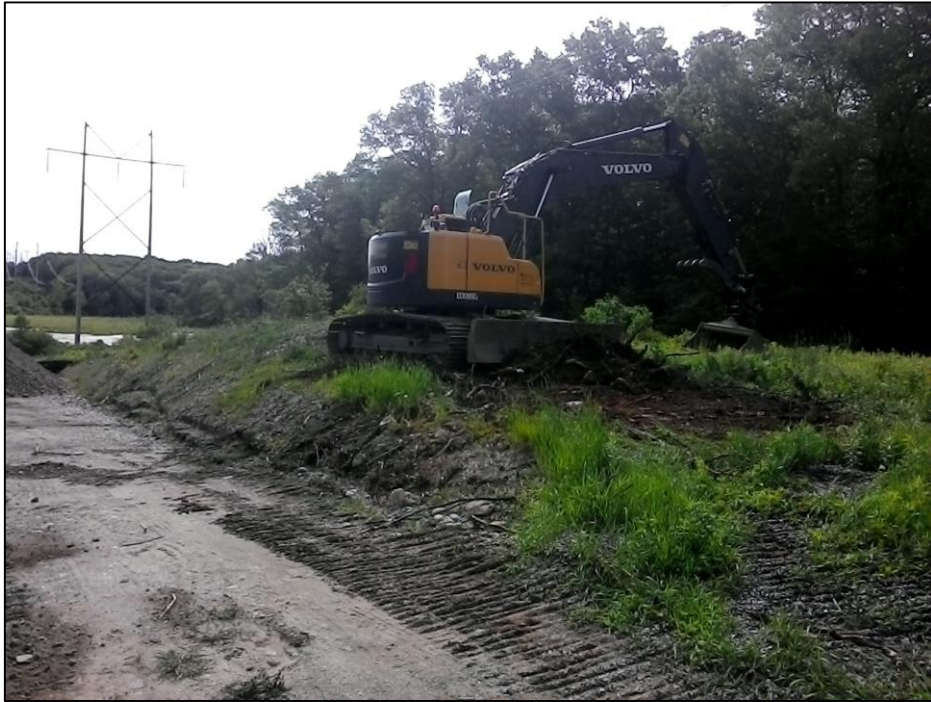
Photo #5: Str 120 pad removal and topsoil spreading as pad of restoration. (6/18)
