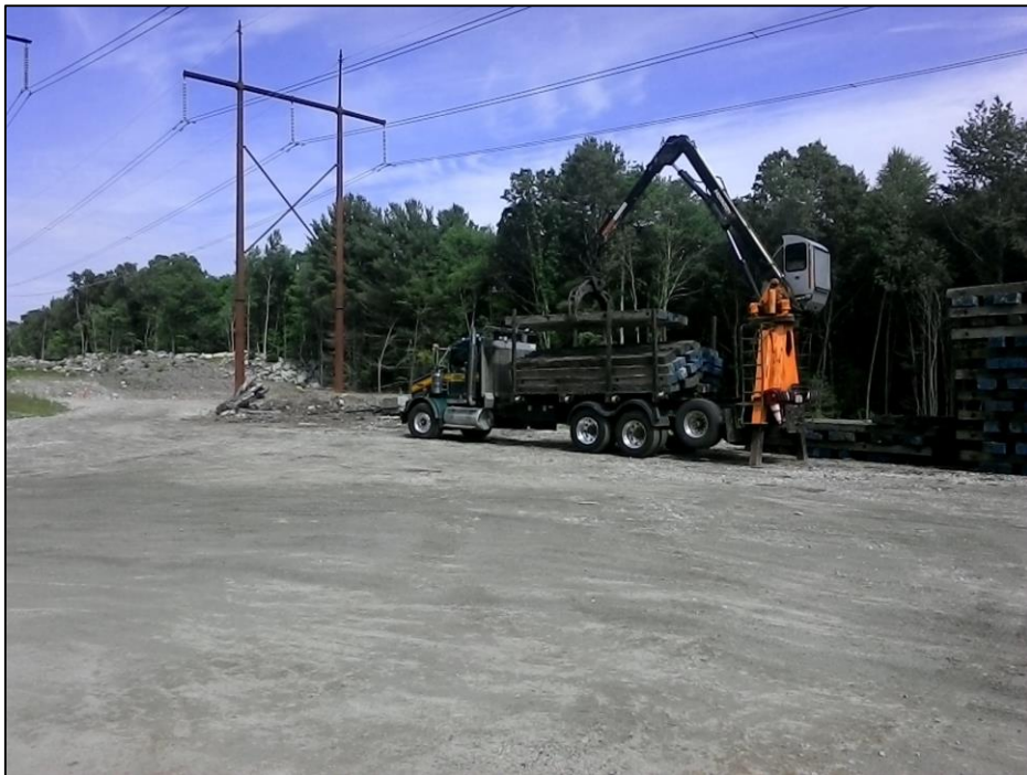
Photo #6: Removing mats at Str 126. (6/18)
