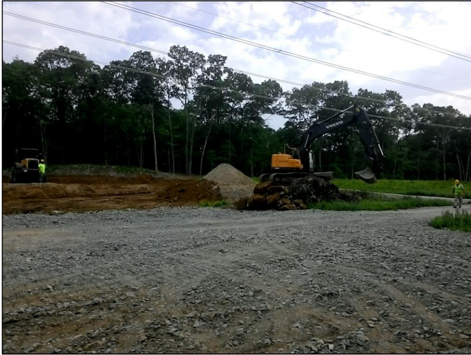
Photo #1: Pad removal as part of restoration at Str 115. (6/11)
