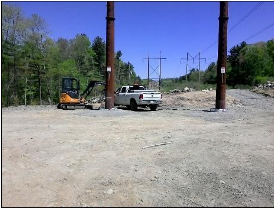
Photo #5: Grounding operations at Str 326. (5/14)
