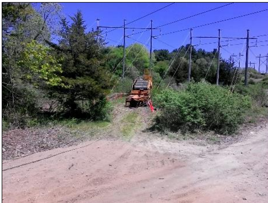
Photo #4: Pulling conductor from Str 241. (5/14)
