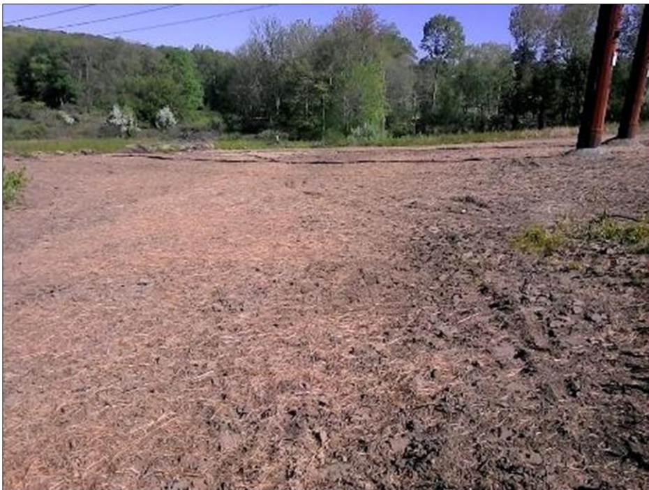
Photo #2: Str 6 seeded and awaiting stabilization. (5/14)
