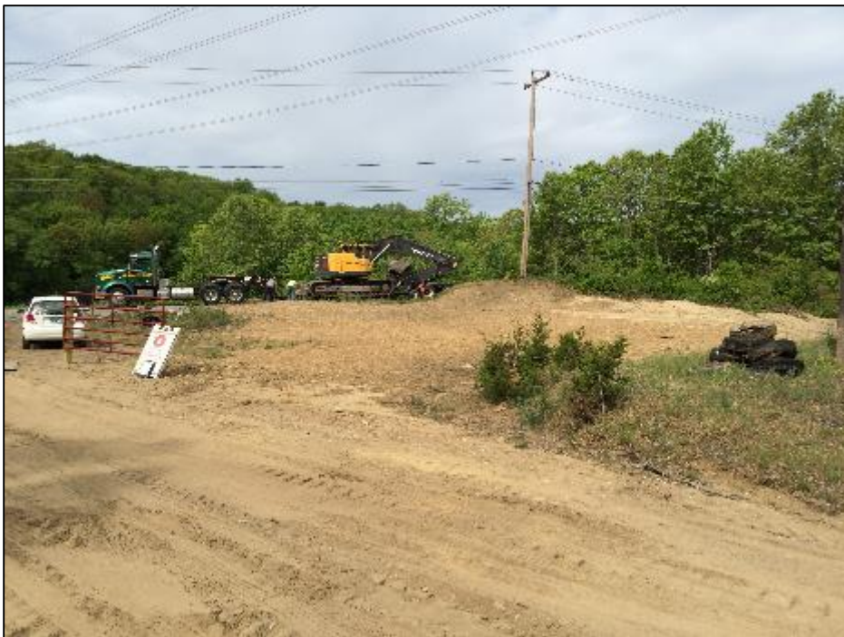
Photo #8: Removal of guard pad at Str 34 as part of restoration (5/21)
