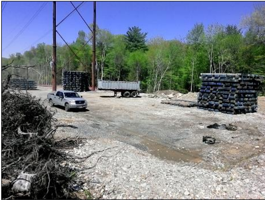
Photo #3: Mat removal and stockpiling at Str 166. (5/14)
