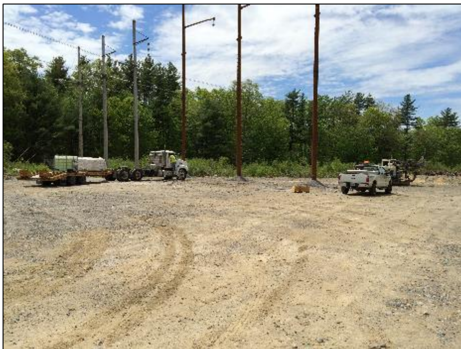
Photo #10: Installation of anchors at Str 325. (5/21)
