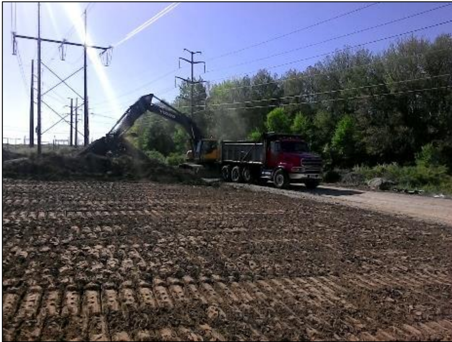
Photo #1: Removing material from Str 3 pad as part of restoration. (5/14)
