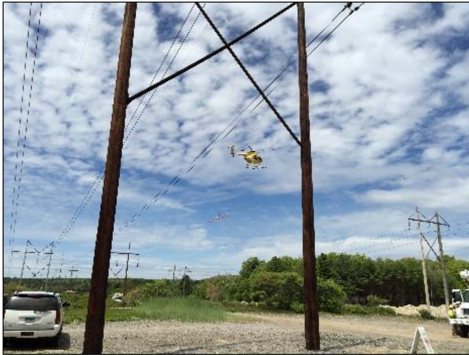
Photo #9: Pulling conductor with helicopter at Str 264. (5/21)
