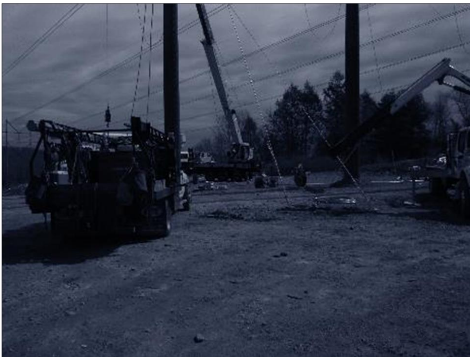
Photo #2: Stringing operations at Str 180. (4/30)
