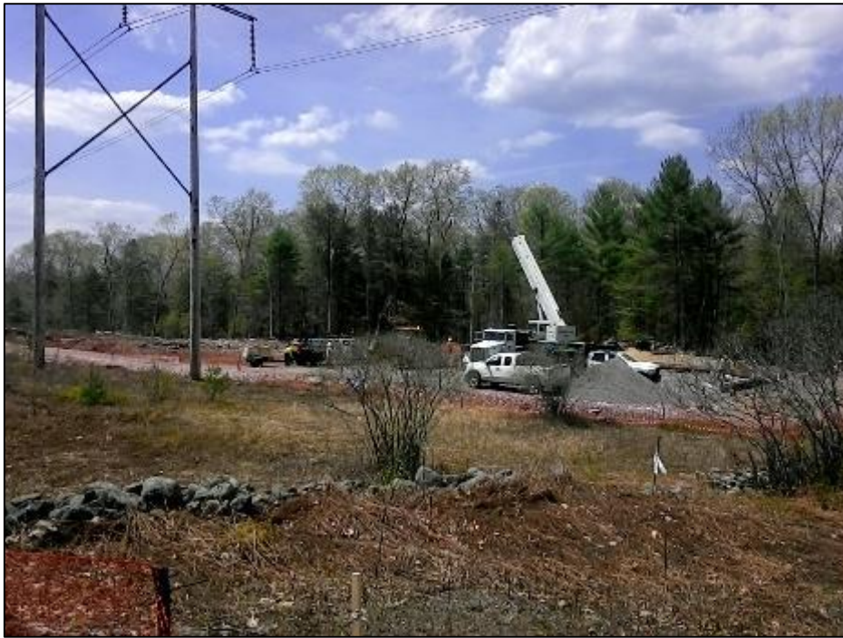
Photo #11: Str 331 erection. (5/8)
