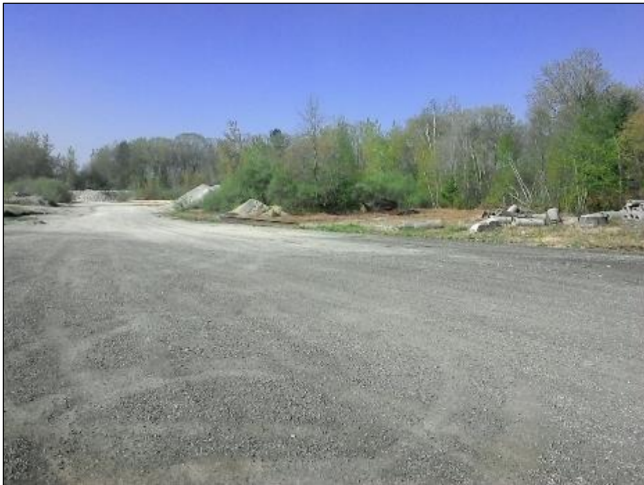
Photo #6: Laydown Yard at Boston Post Road considered stabilized and no longer project-related as of 5/7/15. (5/8)
