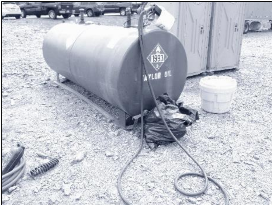
Photo #4: Double-lined 1,000 gallon tank at Nora Lane Laydown Yard. (4/30)
