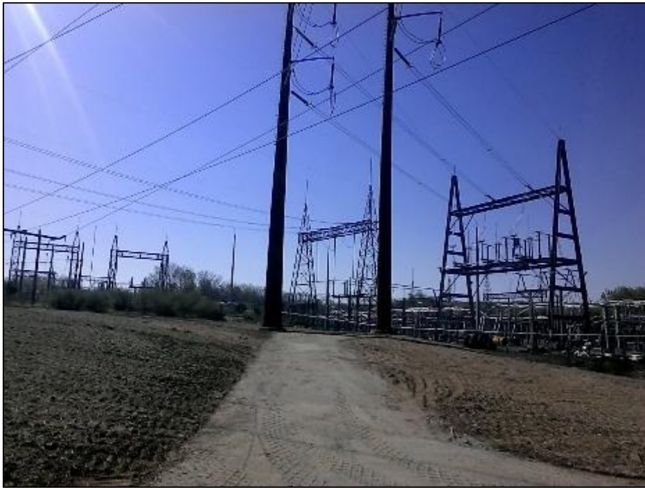
Photo #7: Str 1 pad completely removed and area fully seeded for restoration. (5/8)
