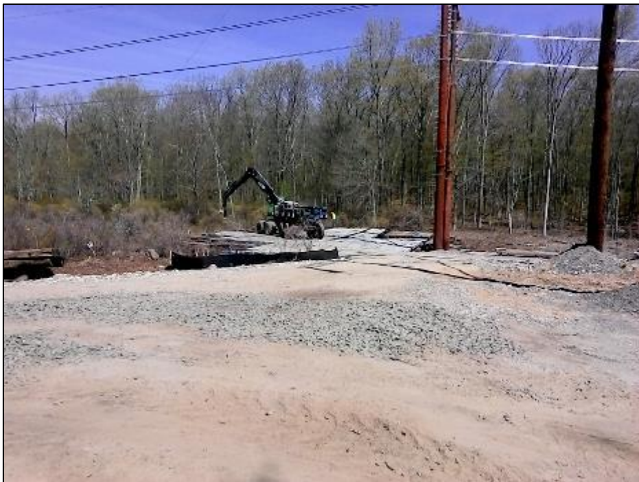
Photo #8: Mat removal at Str 135. (5/8)
