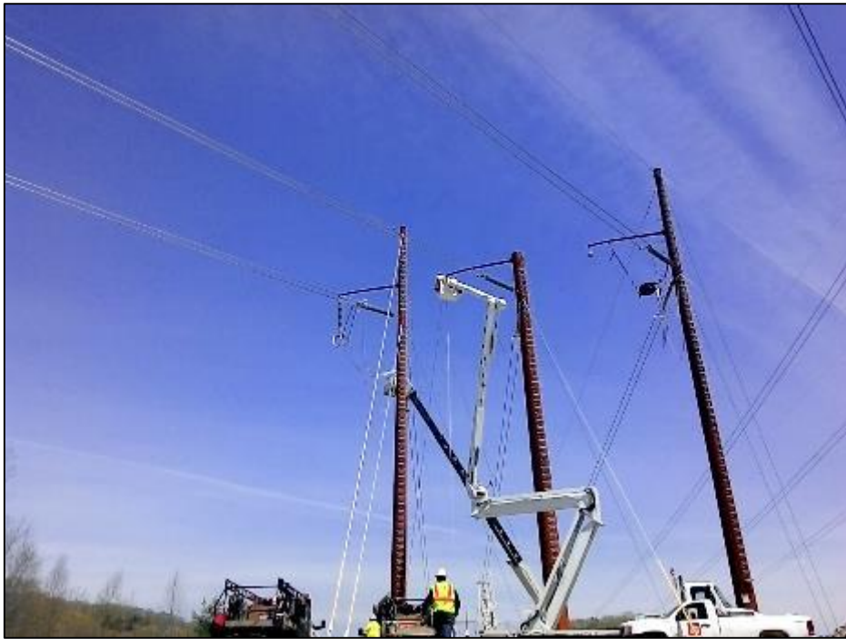
Photo #9: Stringing at Str 204. (5/8)
