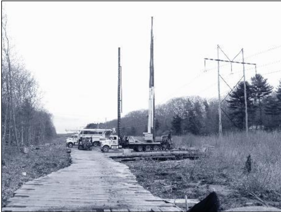
Photo #3: Str 310 erection. (4/30)
