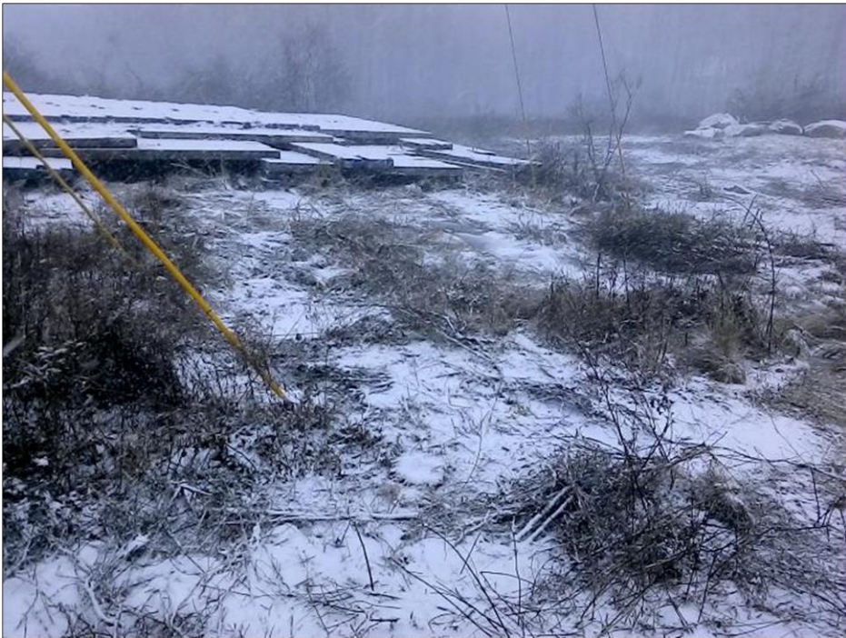
Photo #2: Wetland Mat Removal at Str 15.
