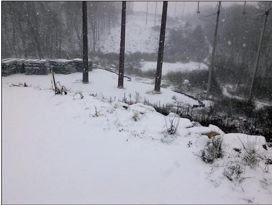
Photo #3: Wetland Timber Mats removed and silt fence installed at Str 49. (1/9)
