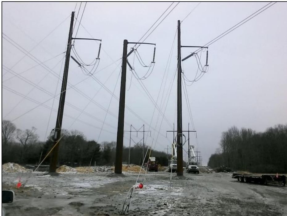
Photo #12: Newly pulled conductor installed to dead-end Str 111. (1/15)
