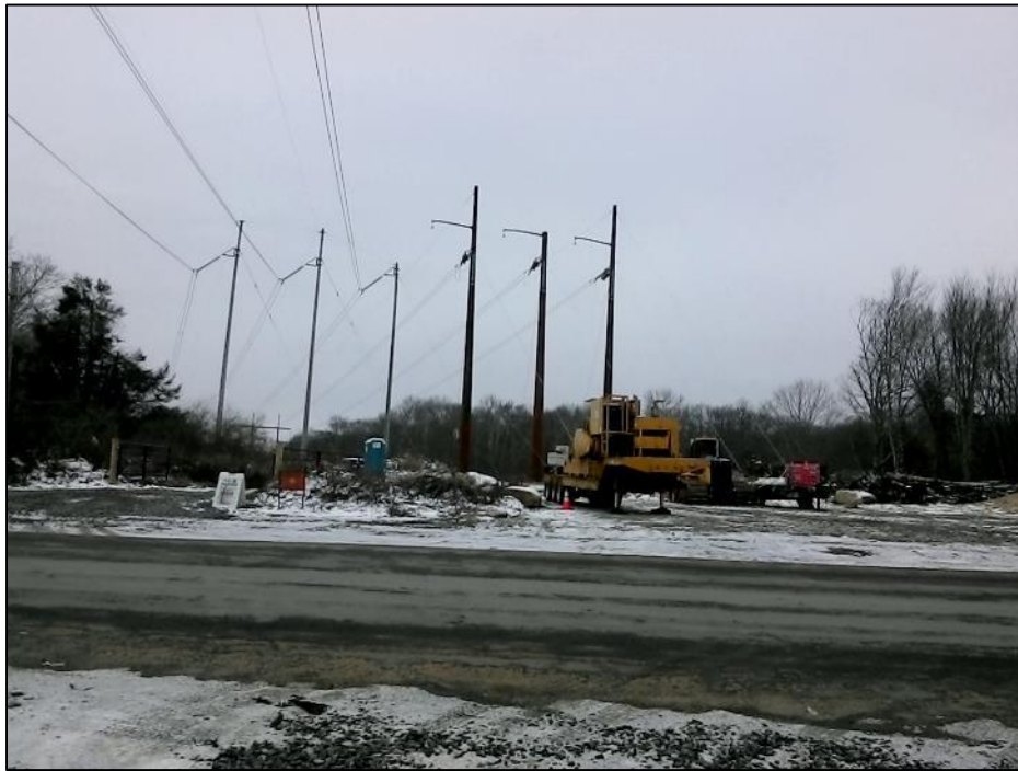
Photo #11: Str 124 pulling area. (1/15)
