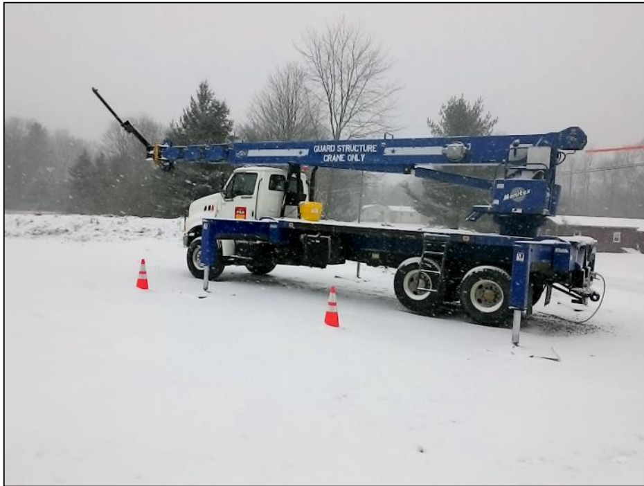
Photo #5: Spill kit visible onsite. (1/9)
