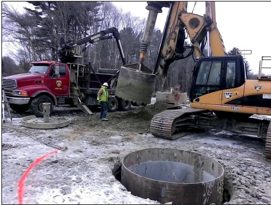
Photo #7: Drilling Operation for Str 293 (1/15)
