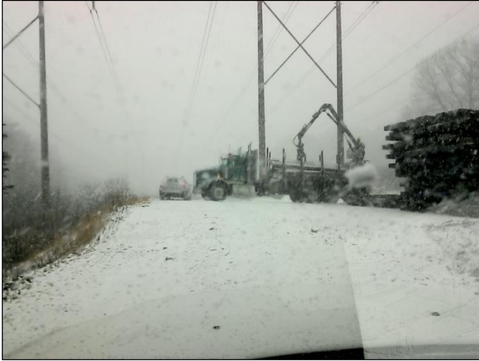
Photo #1: Timber Mat removal in the vicinity of Str 15. (1/9)
