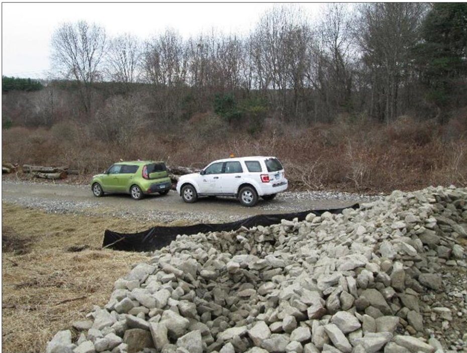
Photo #2: Observed plunge pool and hay bale reinforced silt fence at Str 284. (11/25)
