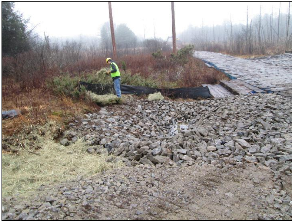
Photo #3: Observed spreading of hay on exposed topsoil at Str 322. (12/3)
