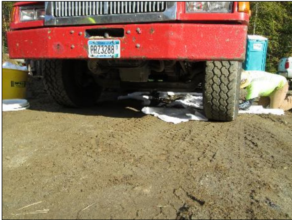
Photo #5: Tri-state crew containing hydraulic fluid spill at Str 49.
