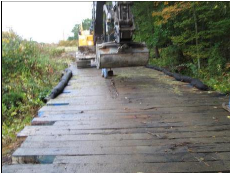
Photo #4: Cleaning of wetland mats up-line of Str 203. (10/1)
