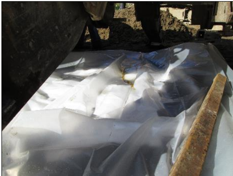
Photo #6: Hydraulic fluid spill contained with plastic and diaper dams at Str 49.
