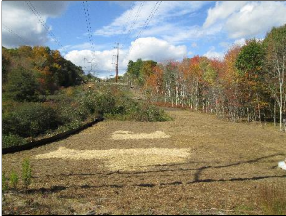
Photo #7: Hay spread over restored topsoil down-line of Str 96.
