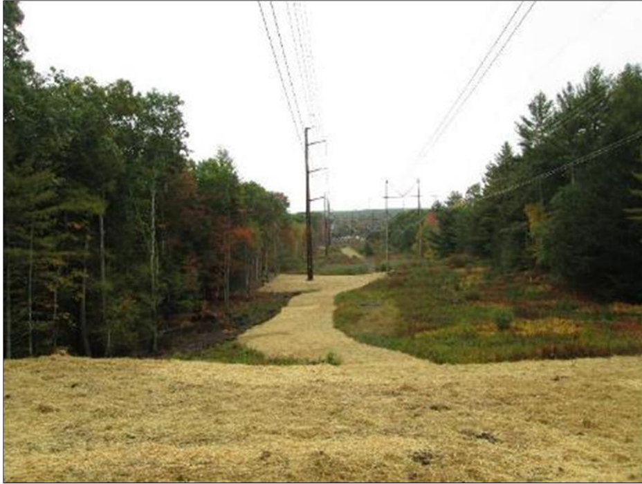
Photo #1: Hay spread over restored topsoil up-line of Str 97. (10/1)
