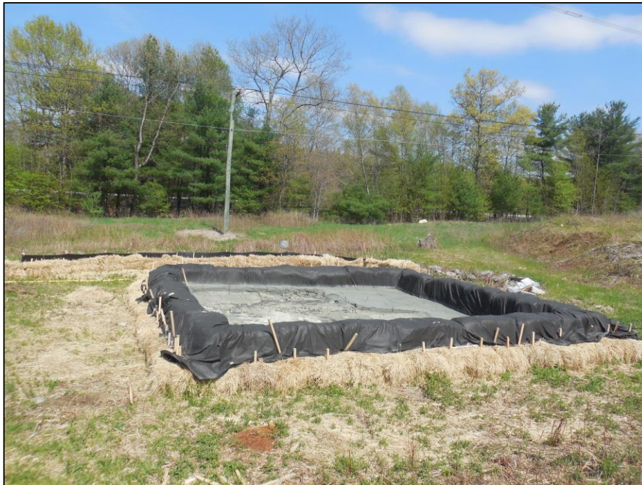
Photo #8: (5/14) Concrete wash out area up-line of Str 265.
