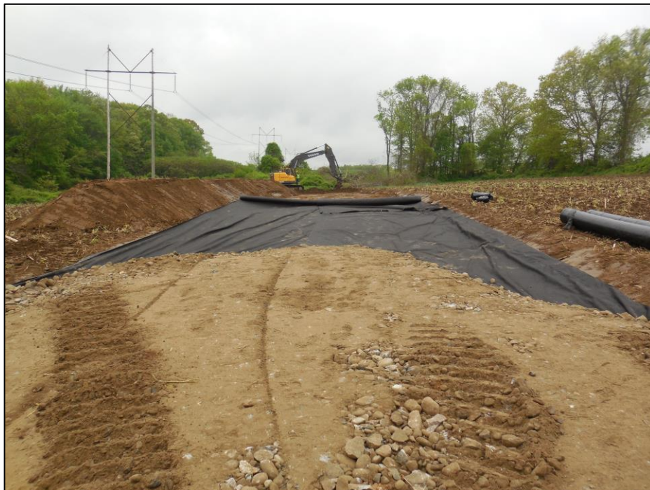
Photo #6: Access road in agricultural farmland area being installed with filter fabric barrier up-line of Str 53.
