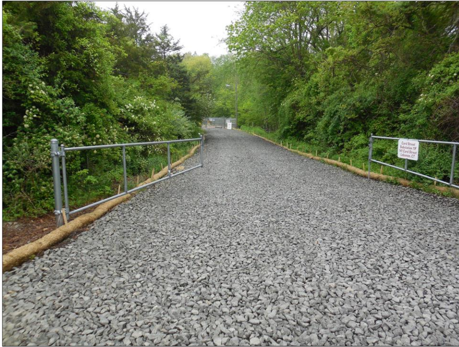
Photo #1: View of entrance pad at CSSS.
