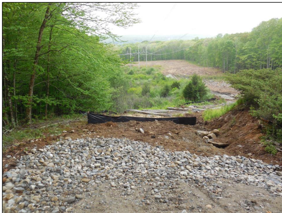
Photo #4: Photo of erosion control measures down-line of Str 43.
