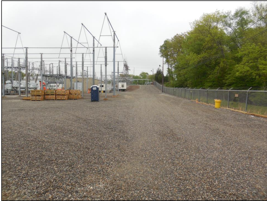
Photo #3: Area where new stone that was placed at CSSS.
