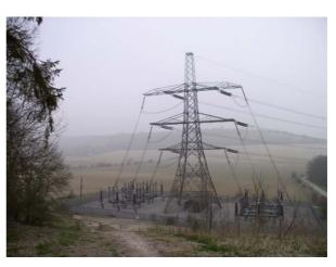
Transition stations are used to connect lines and cables together
