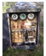
Kiosk containing pressure gauges and fluid leak alarms
