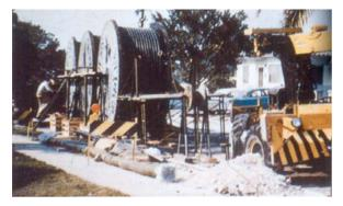
Three reels of cable are parked in the street ready to be pulled into a steel pipe
