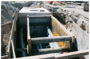
Ducts entering a single, pre-cast concrete splicing vault
