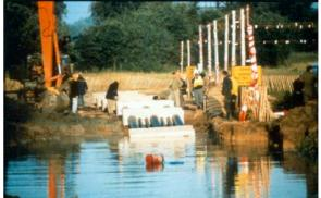
Installation of ducts to house the cables that will cross the river
