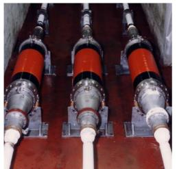
Joints near completion in a joint bay, they will later be buried with soil up to street level
