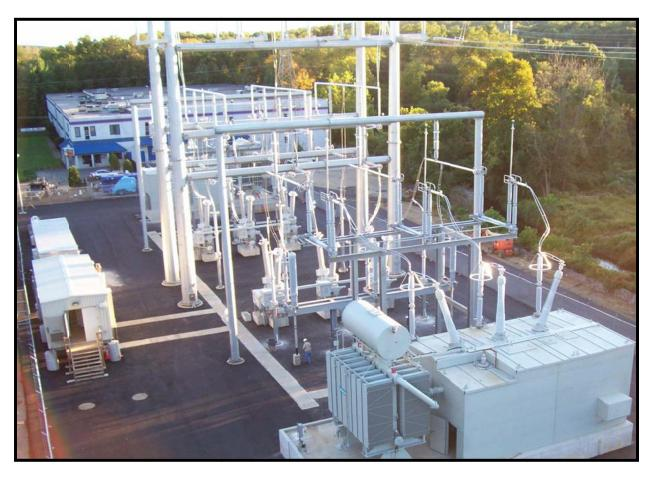
Figure 15A-2: 345-kV Line Transition Station with Shunt Reactors
