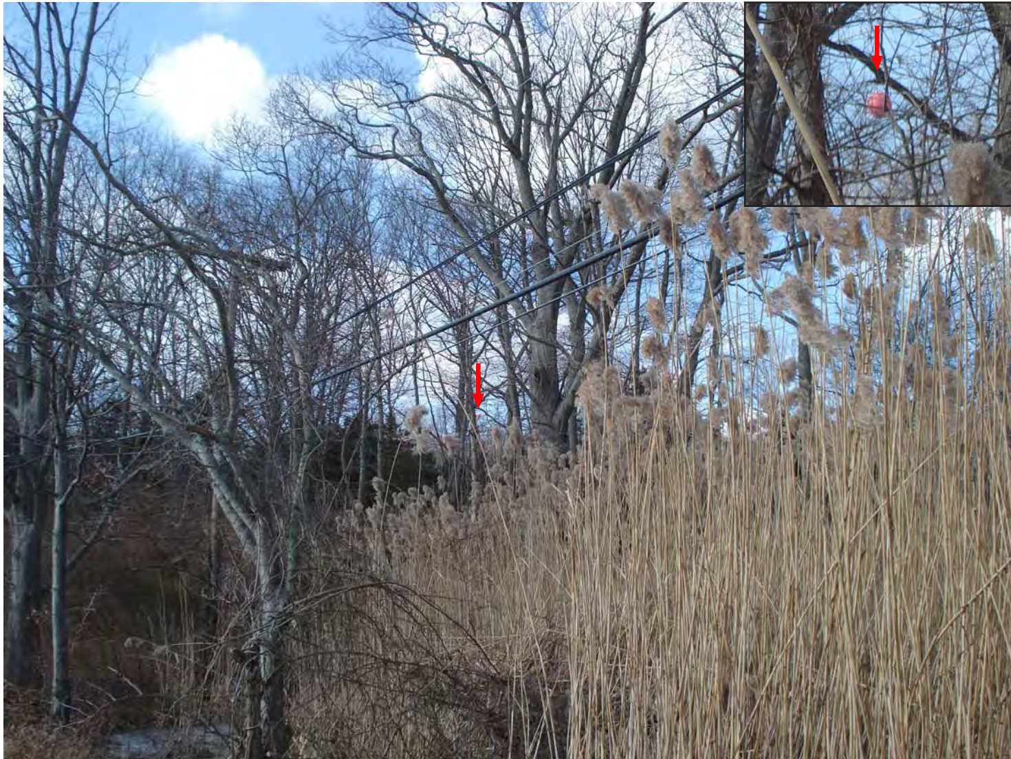
Photosim for conceptual purposes only - actual antenna & equipment locations to be determined based on final engineering design
