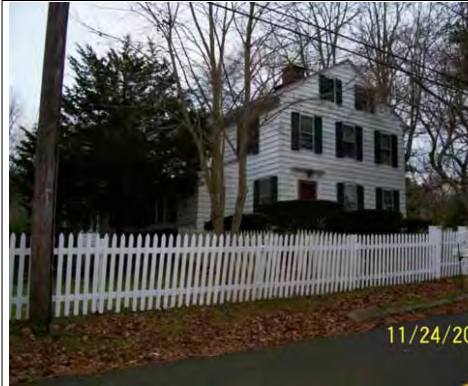
15. Facing northwest toward 133 Moose Hill Road.
