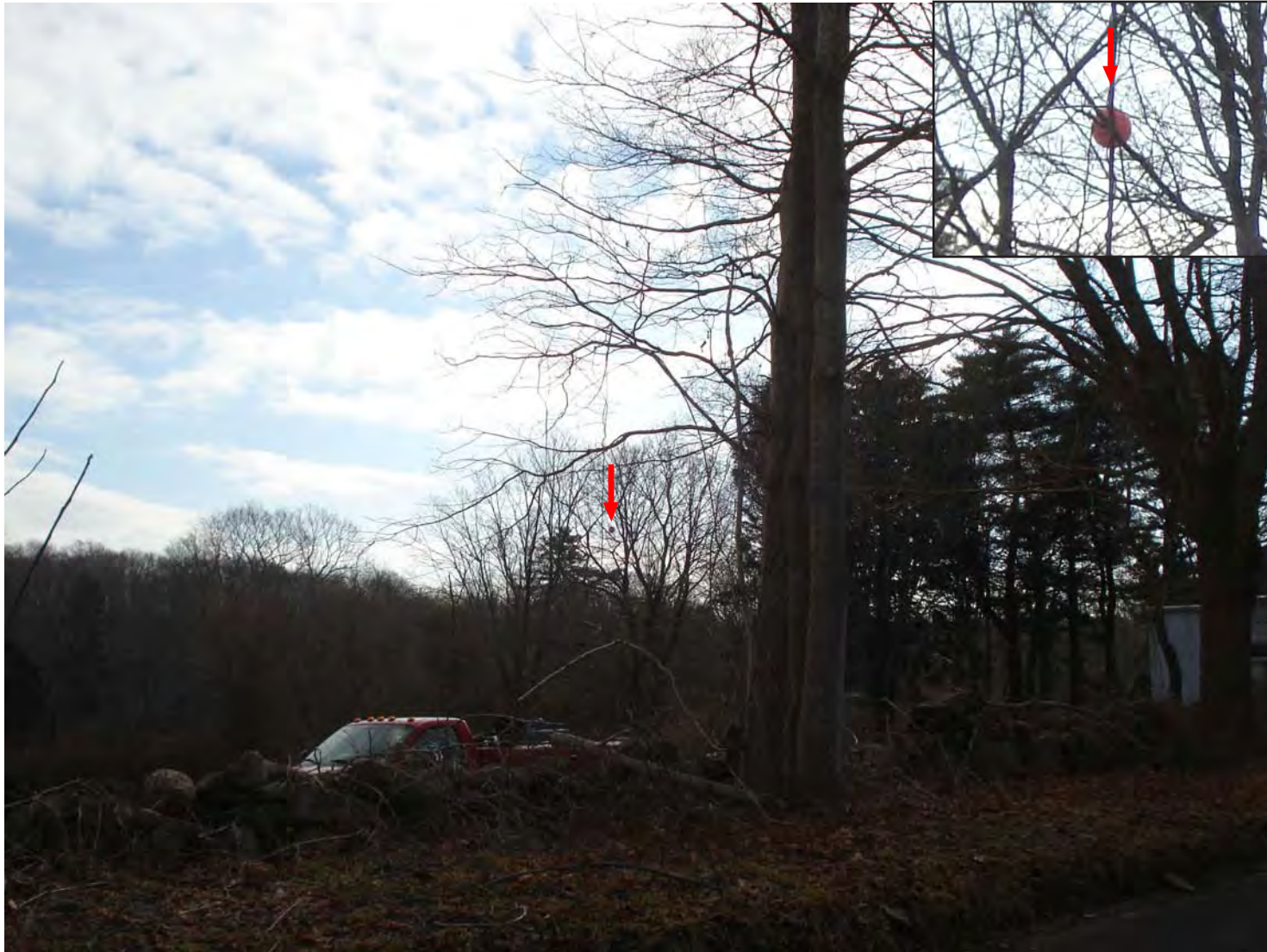
Photosim for conceptual purposes only - actual antenna & equipment locations to be determined based on final engineering design
