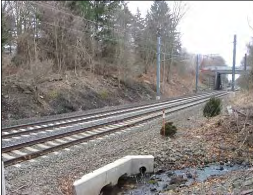
13. Facing southwest toward Amtrak railroad from the existing gravel access drive.
