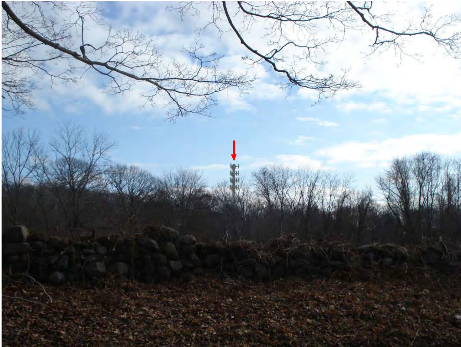
Photosim for conceptual purposes only - actual antenna & equipment locations to be determined based on final engineering design
