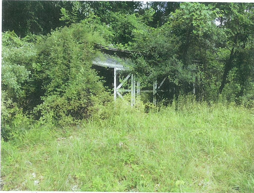
Photo 3: View of small dilapidated shed in northwest corner of proposed alternate Site, looking north.
