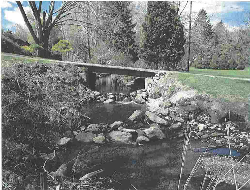
Photo 15: View of driveway bridge over Wewaka Brook (Wetland 5), looking north. (04/19/10)
