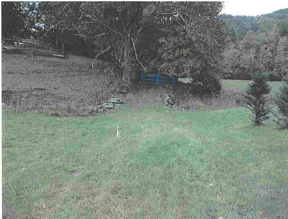
Photo 13: View of farm road crossing of Wetland 4, looking east. (10/05/10)
