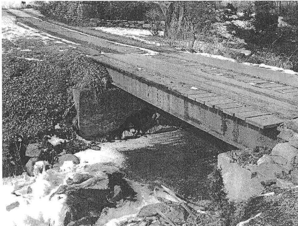
Photo 1: Existing Bridge Structure Across Wewaka Brook
