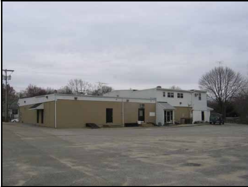
Photo 5: View facing northeast of the rear of the existing commercial building on the Subject Property (note existing utility pole at left)
