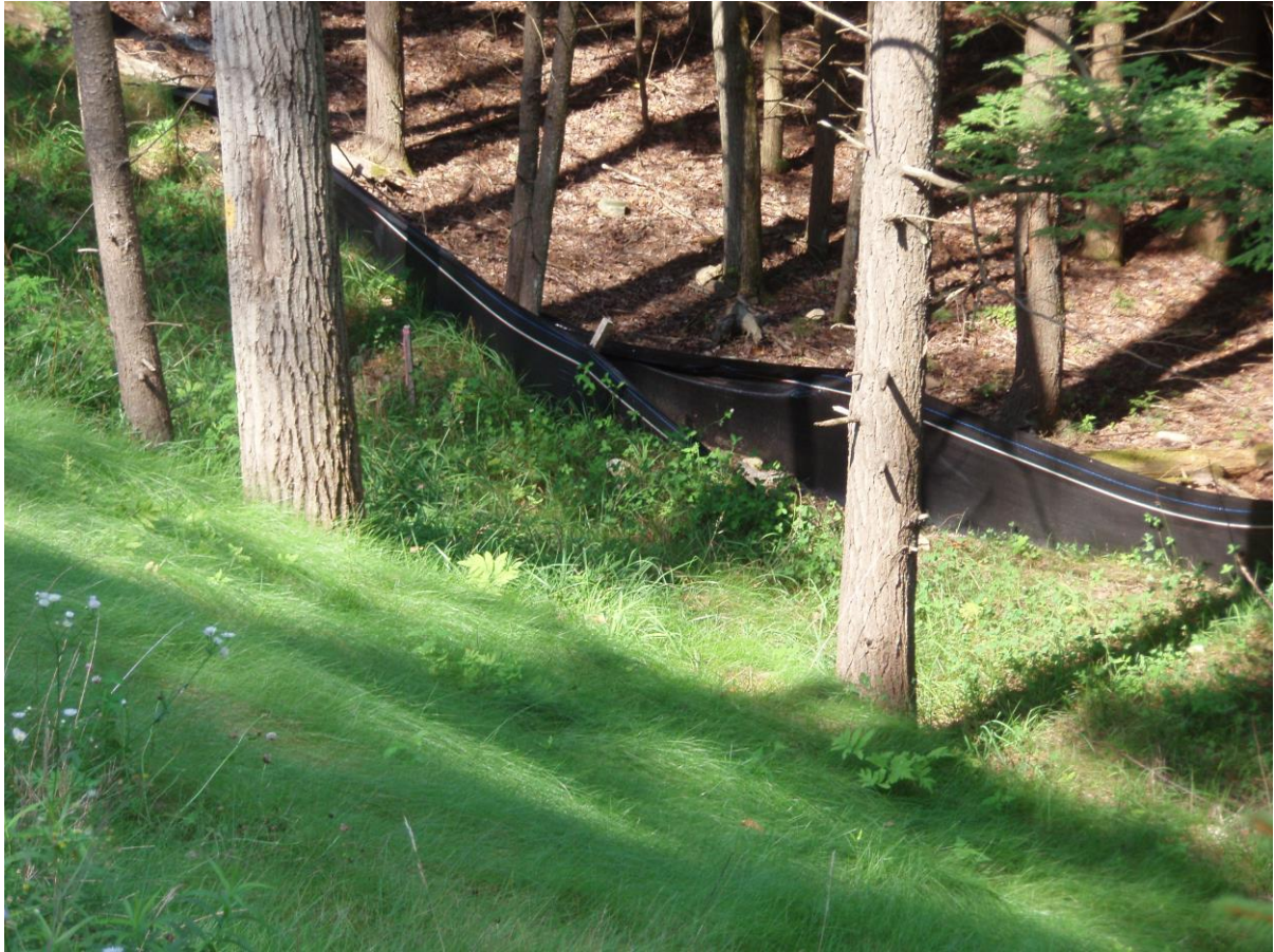
Erosion control fence at base of re-vegetated embankment.
