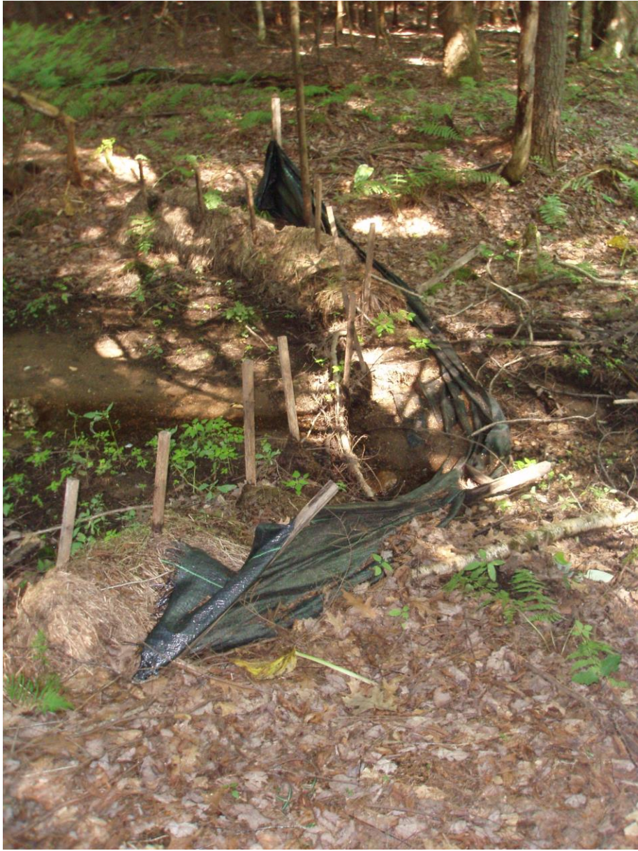
Erosion control fence in wetland area north of bridge.
