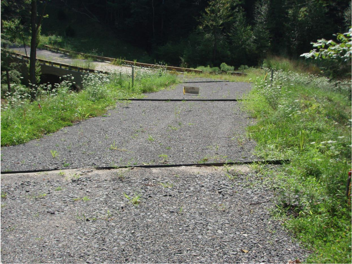
Rubber deflectors in the access road. Note re-vegetated side slopes.
