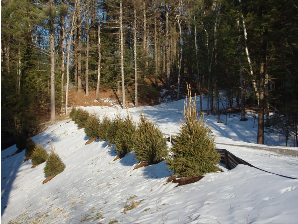
Docket 380: Access road embankment
