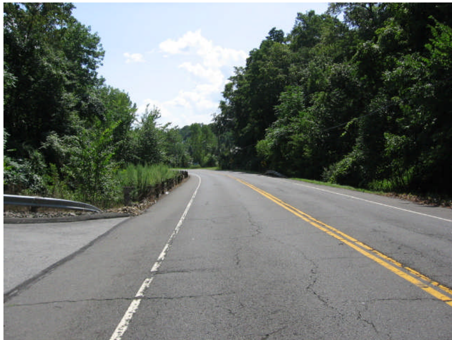
Route 71 Looking South
