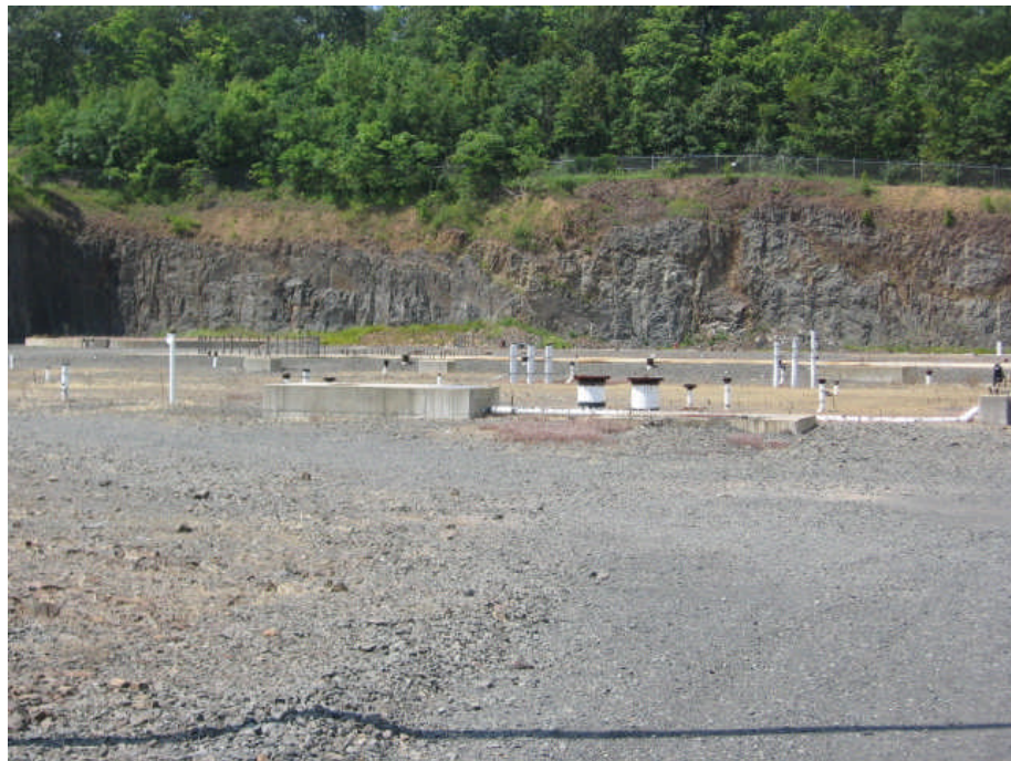
Piping and support for equipment that was removed on west side of main building
