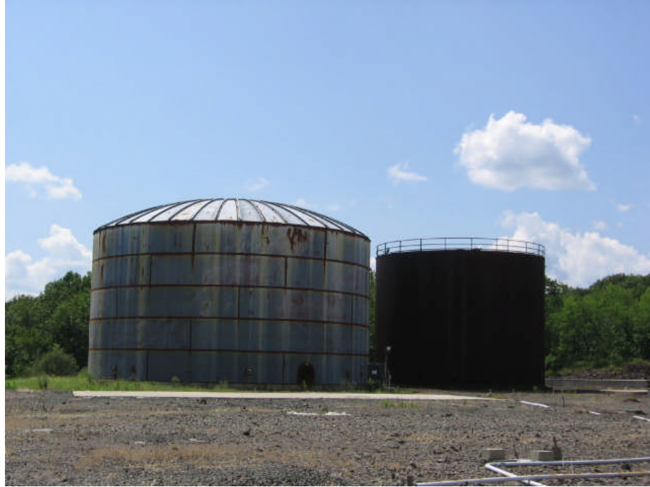
Above ground Water and Fuel Tanks
