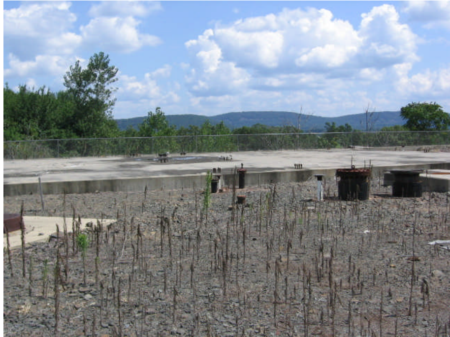
Foundation east of control-administration building
