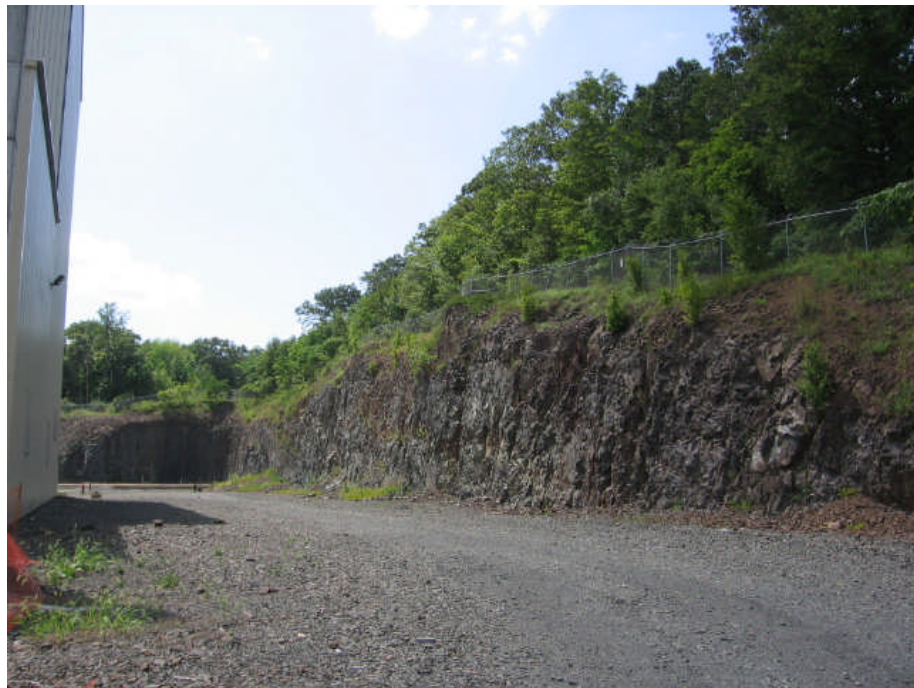
Site north of power plant looking west at rear of power plant building
