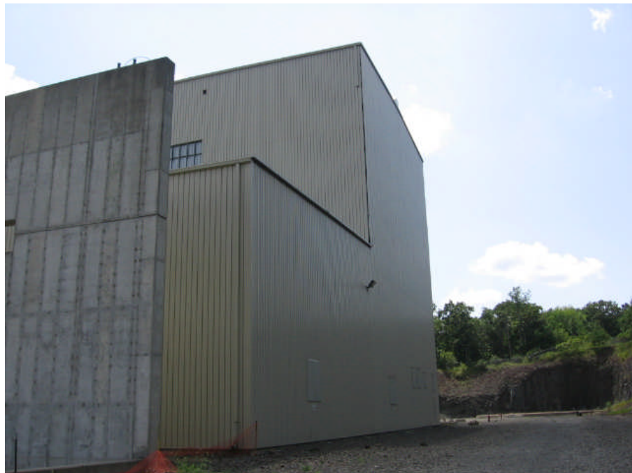
Rear (north side) view Looking West
