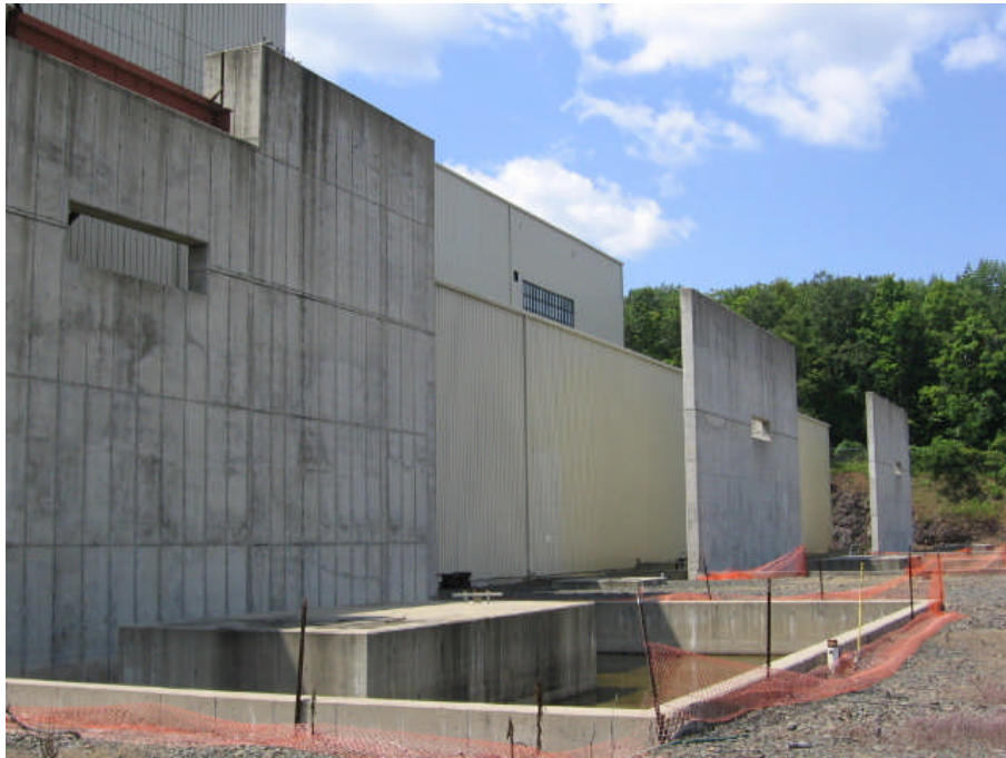
East side looking north
