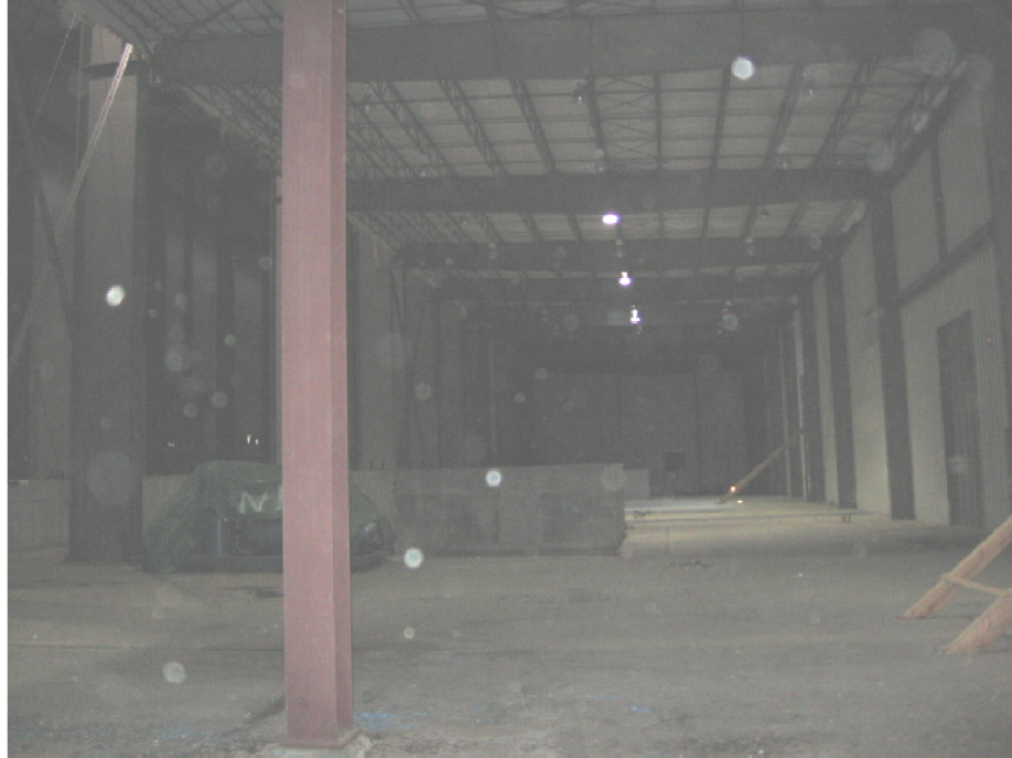
Power Plant Interior view looking to north end
