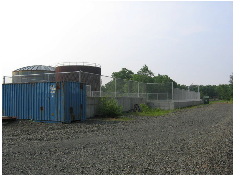
Foundation for Cooling Tower
