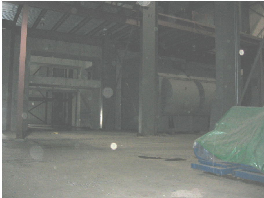
Power Plant Interior View Looking to south end of building
