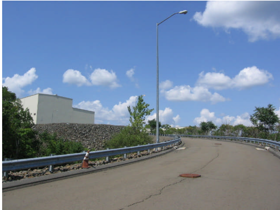
Access Road Looking to Power Plant
