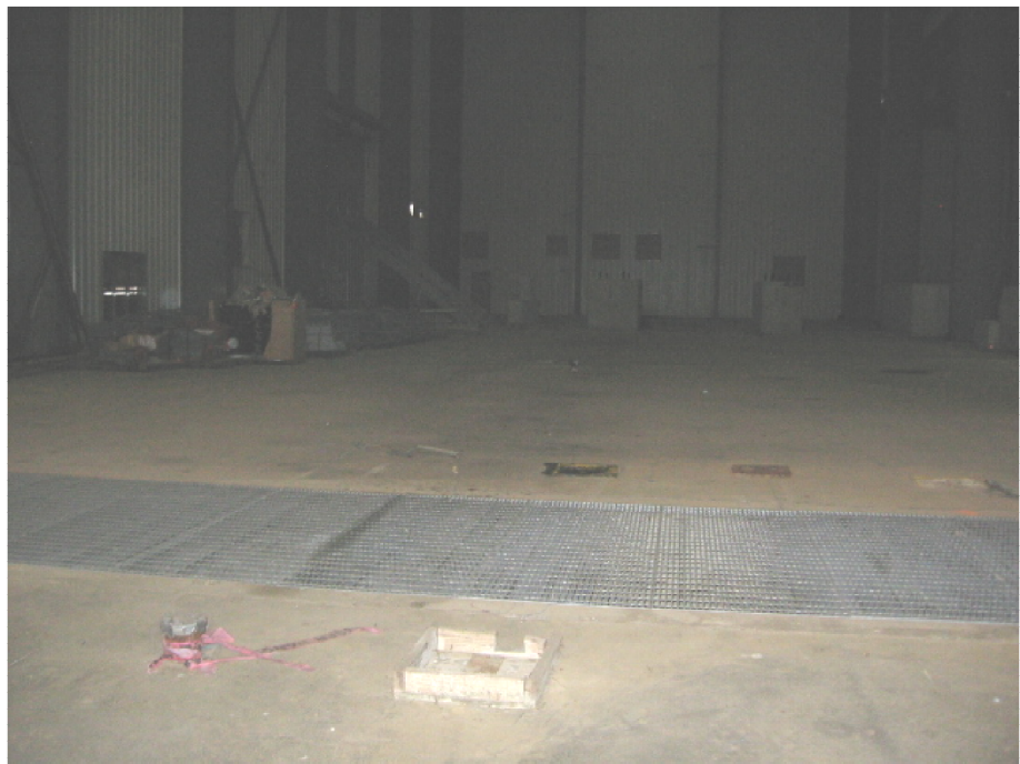
Power Plant Interior view
