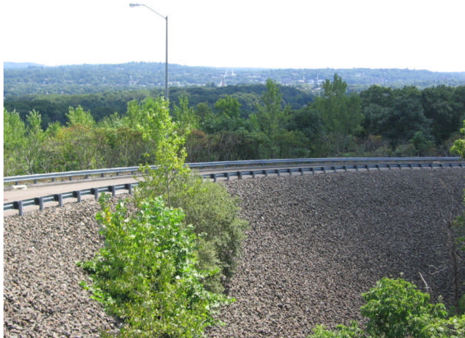
Slope on side of access road and view to south
