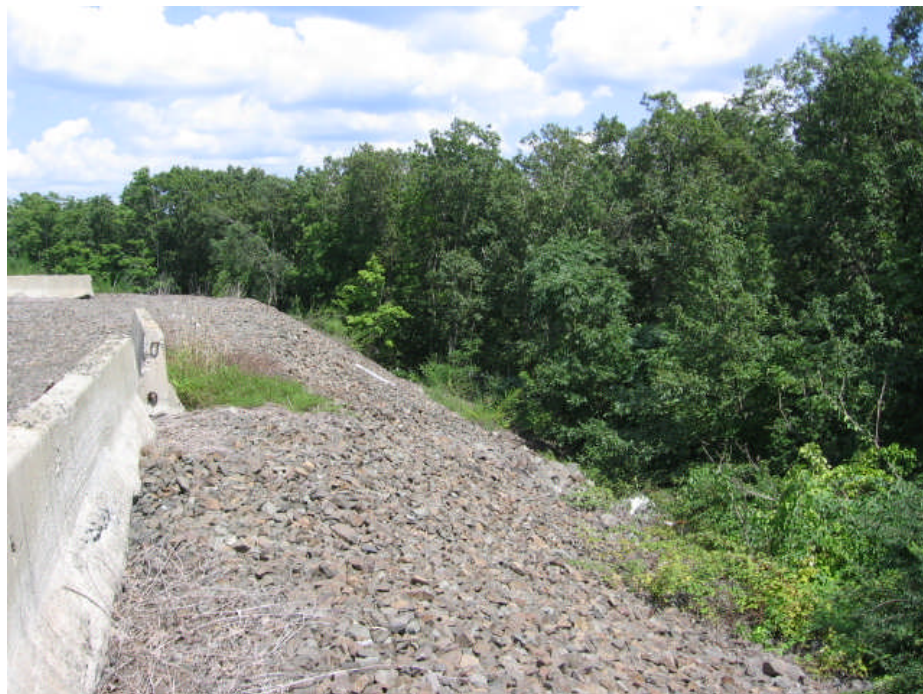
Slope on east side of site
