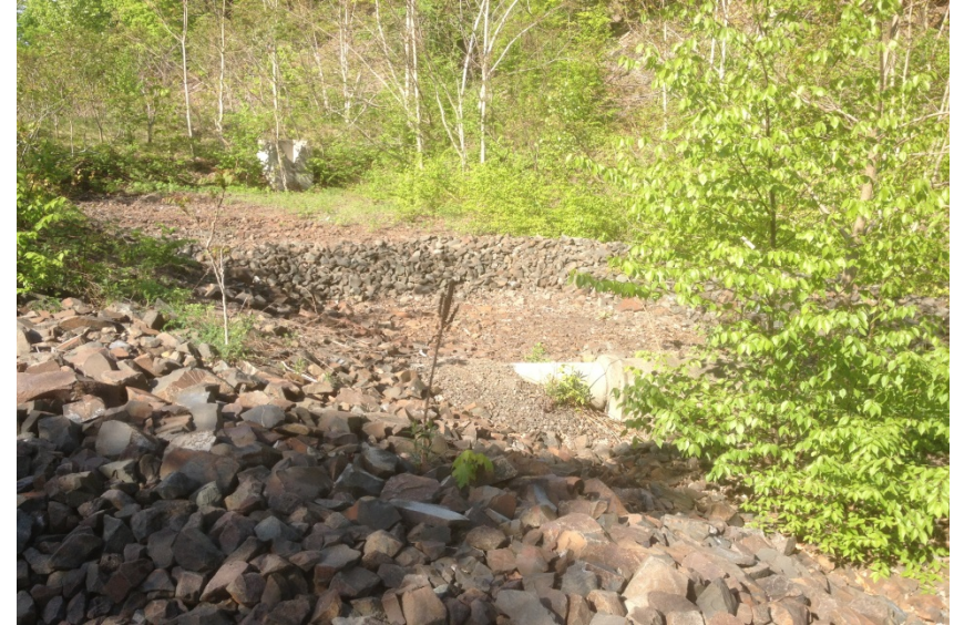
Photo of detention pond with no vegetation established.
