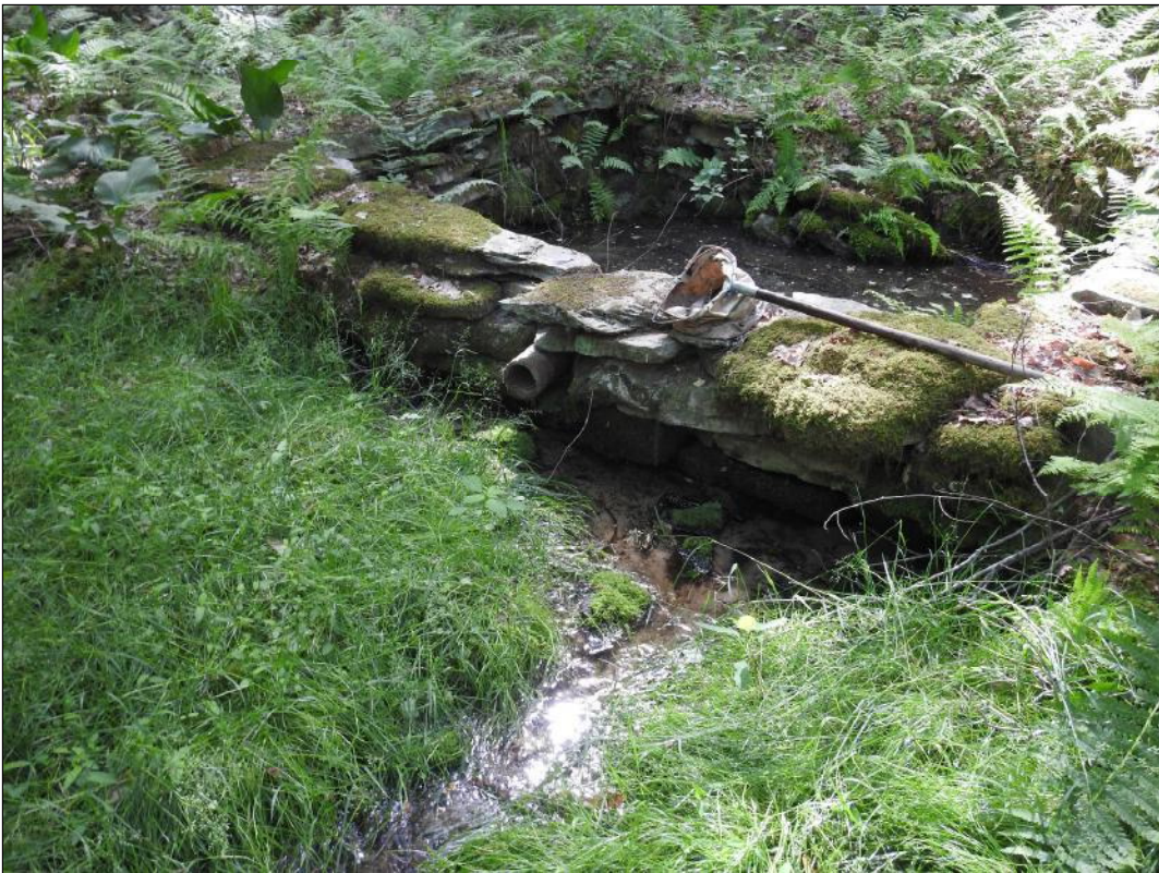
Photo A3-4: Wetland A3, cistern at wetland's spring; 6-10-16; facing easterly
