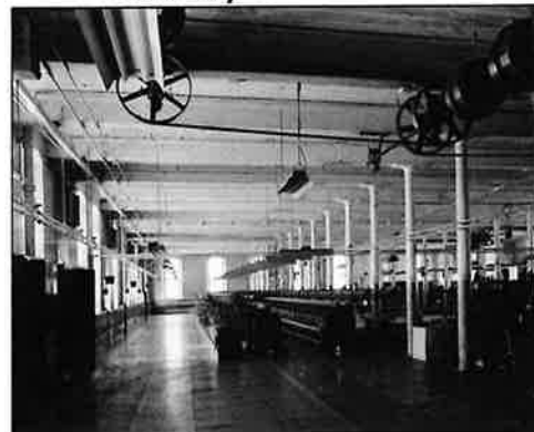
Machinery At Ponemah Mill
