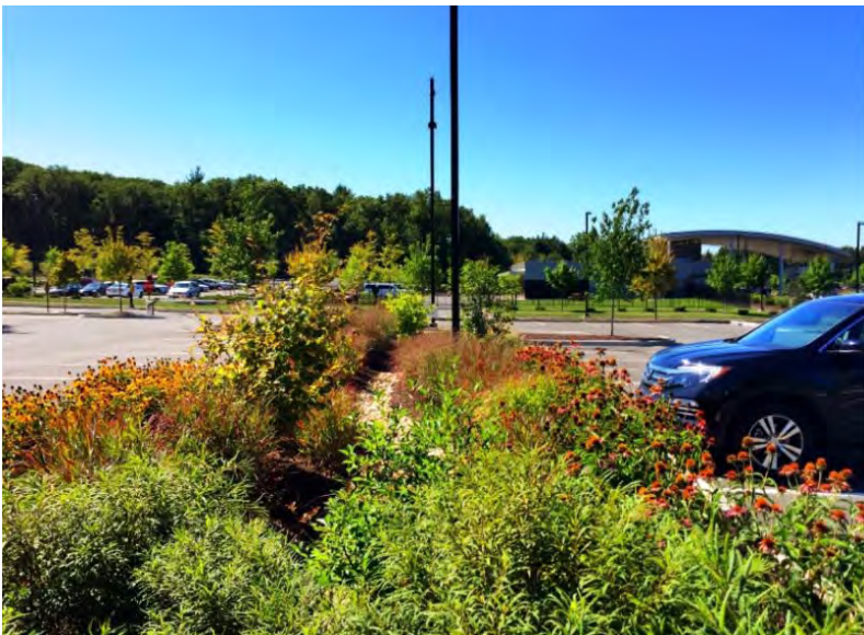
Left: Parking lot rain garden to absorb runoff at ESPN Headquarters in Bristol
