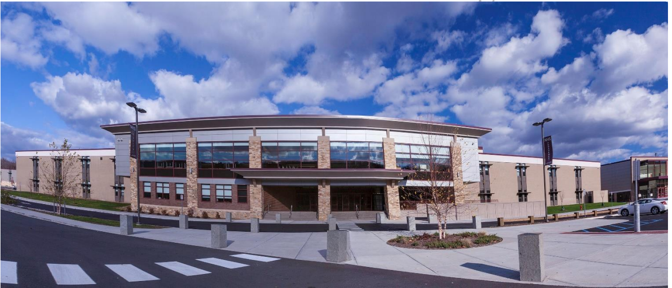
Source, O&G Construction, Newly Renovated Naugatuck High School
