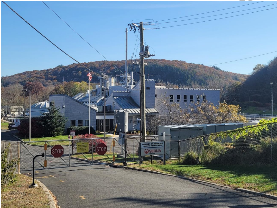
Veolia Water Treatment Plant
