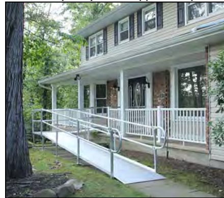
Temporary Handicapped Ramp
