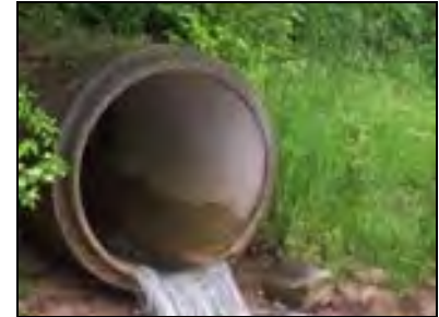
Typical Drainage Outlet
