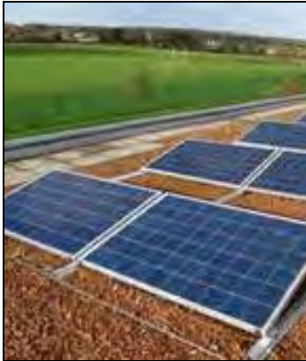
Rooftop Solar Installation
