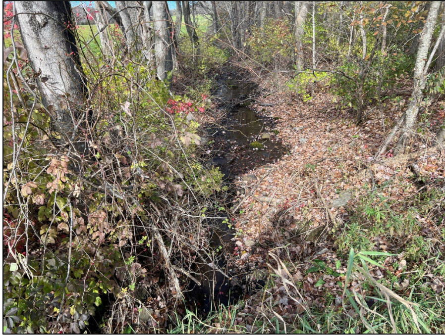
Photo 3: View north of Wetland 1 from culvert inlet headwall at Upper Road.
