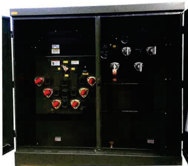
Fig 2. Three Phase Maddox Padmount Transformer
