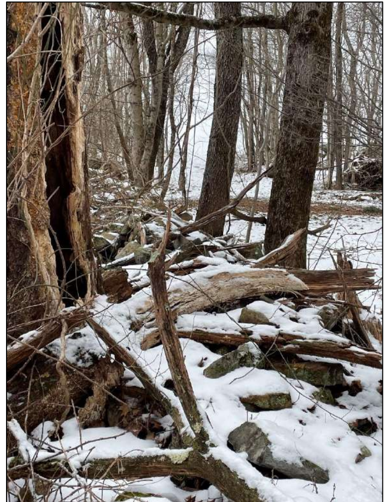
Photo 18. Overview of stone wall. Photo taken facing west.
