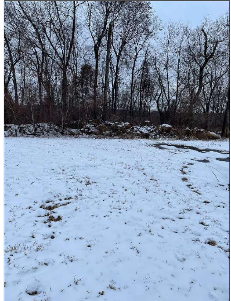
Photo 20. Overview of stone wall from northwest corner of project area. Photo taken facing west.
