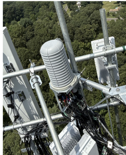
Tower top surge suppressor installed
