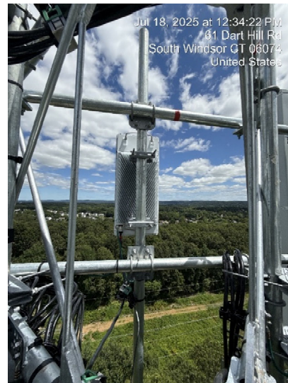
Installed AT&T Air6472 antenna
