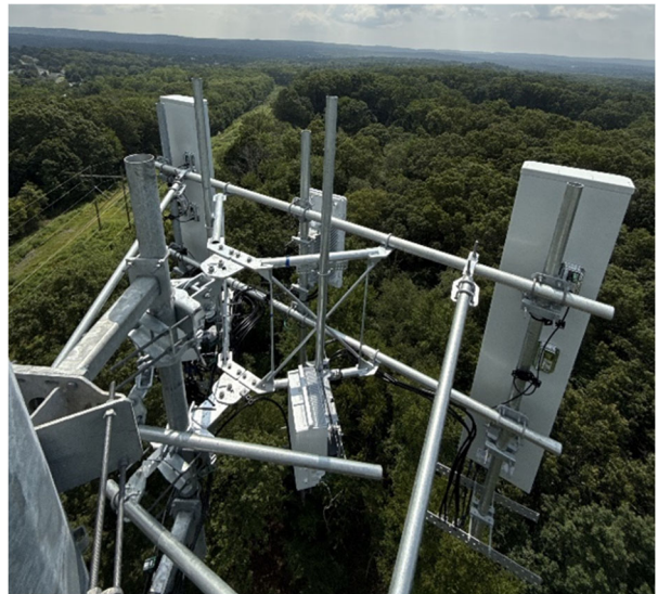
Typical AT&T sector frame installation with tiebacks
