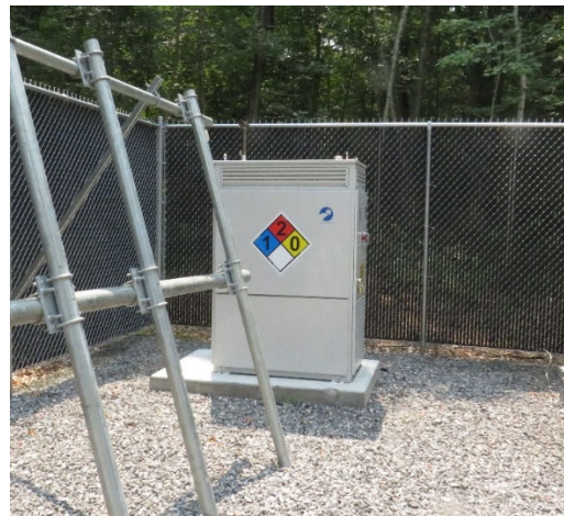
Generator with emergency disconnect
