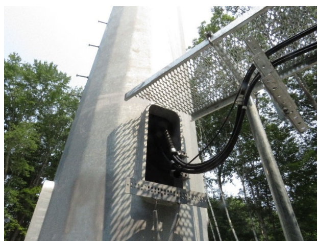
Fiber & DC cables installed and grounded
