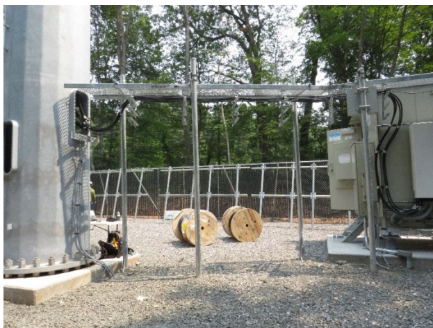
Ice Bridge installed
