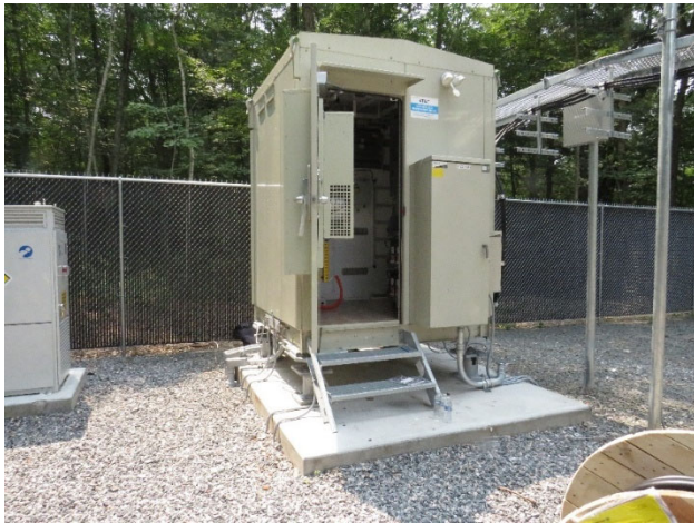
AT&T walk-in equipment cabinet
