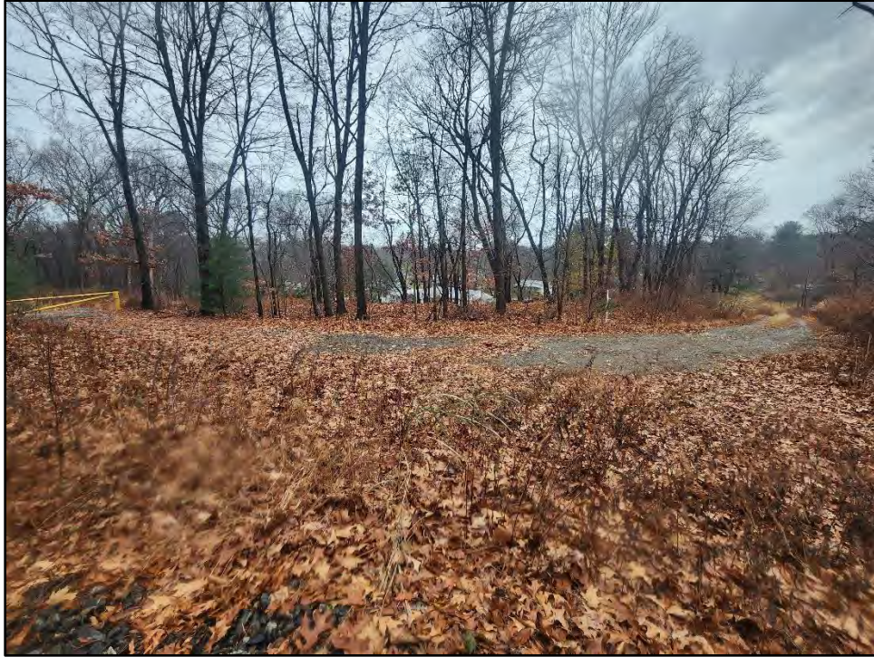
Photo 7. Overview photo from northern end of existing gravel access road location. Photo taken facing west.
