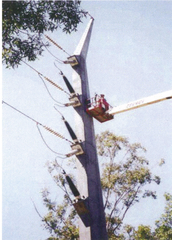
Figure 5. 110 kV single circuit vertical transition tower from OH to UG with well positioned surge arresters. (Courtesy of Powerlink) [2]
