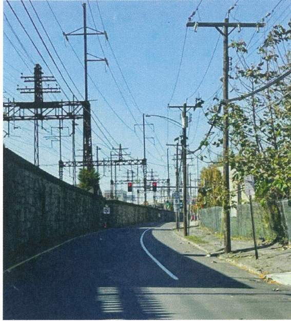
Figure 16. Underground cable route with easy road access. Distribution line (right) could be installed in the duct system.
