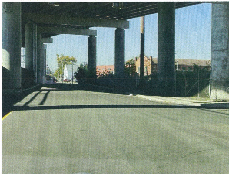
Figure 17. Underground cable route under the highway eliminating the need for very high OH line monopole towers. (see Figure 13)
