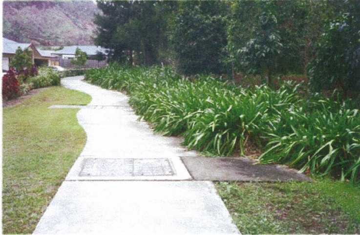
Figure 7. 275 kV XLPE cable installation under pathway through a residential area. (OCEI).
