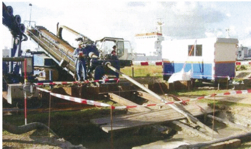
Figure 4. HDD (Horizontal Directional Drilling) [2]
