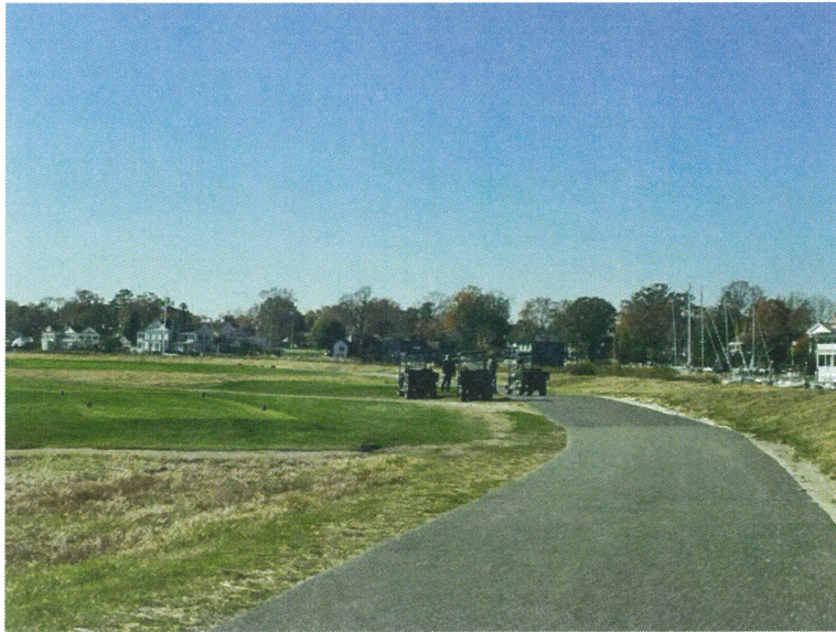
Figure 21. Modified route along the golf course road reducing route length and allowing HDD access under Southport Harbor.
