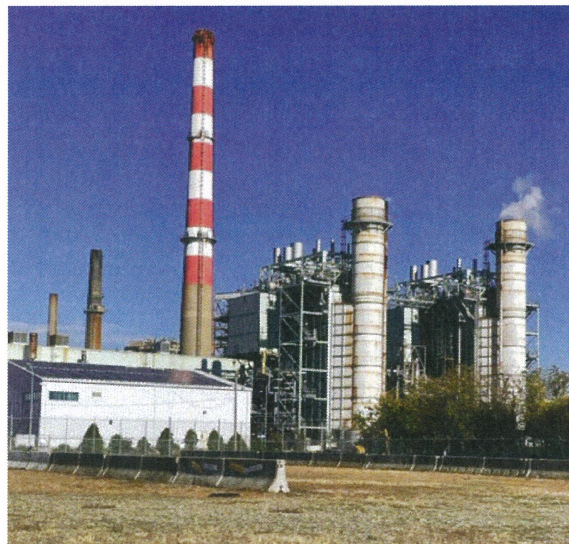
Figure 9. Bridgeport generation plant.
