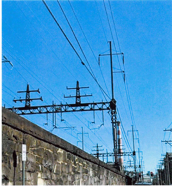
Figure 14. Railway overhead catenary and bonnet construction.
