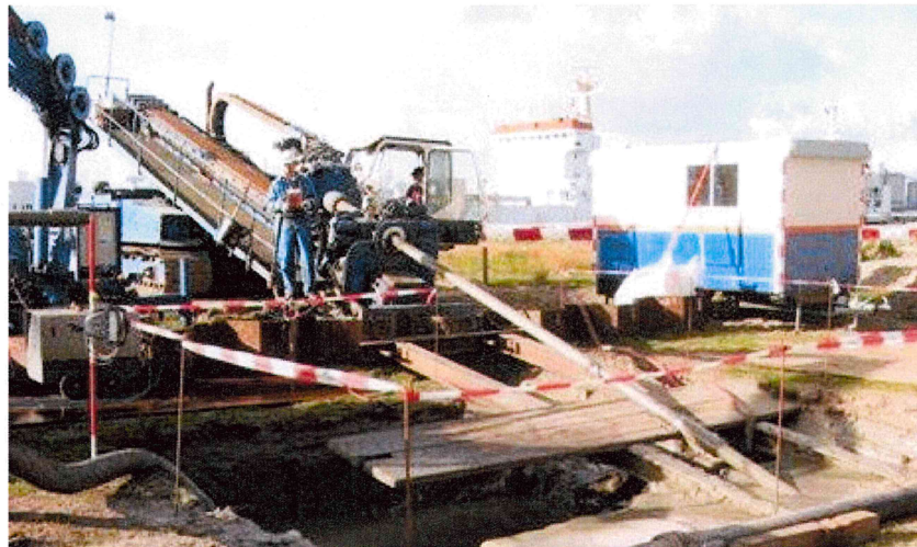
Figure 4. HDD (Horizontal Directional Drilling) [2]
