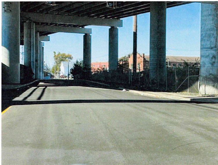
Figure 17. Underground cable route under the highway eliminating the need for very high OH line monopole towers. (see Figure 13)
