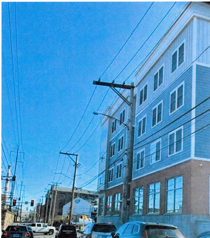
Figure 15. Dangerous OH line installation close to offices and apartments.
