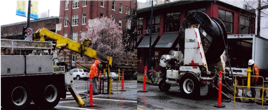
Figure 3. Underground cable upgrading program in a duct system, pulling (left) and cable feed (right). (Courtesy of BC Hydro/OCEI) [2]
