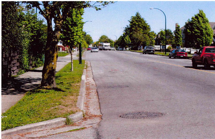
Figure 6. In-road installation of a 138 kV transmission cable. Only the manhole covers are visible. (OCEI)
