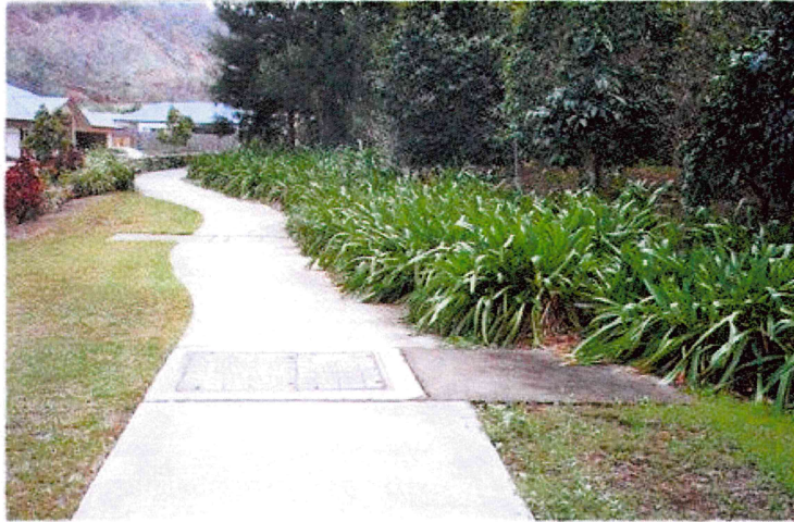
Figure 7. 275 kV XLPE cable installation under pathway through a residential area. (OCEI).
