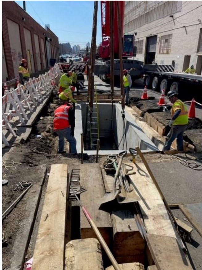
Figure 5. Placing a precast concrete manhole.
