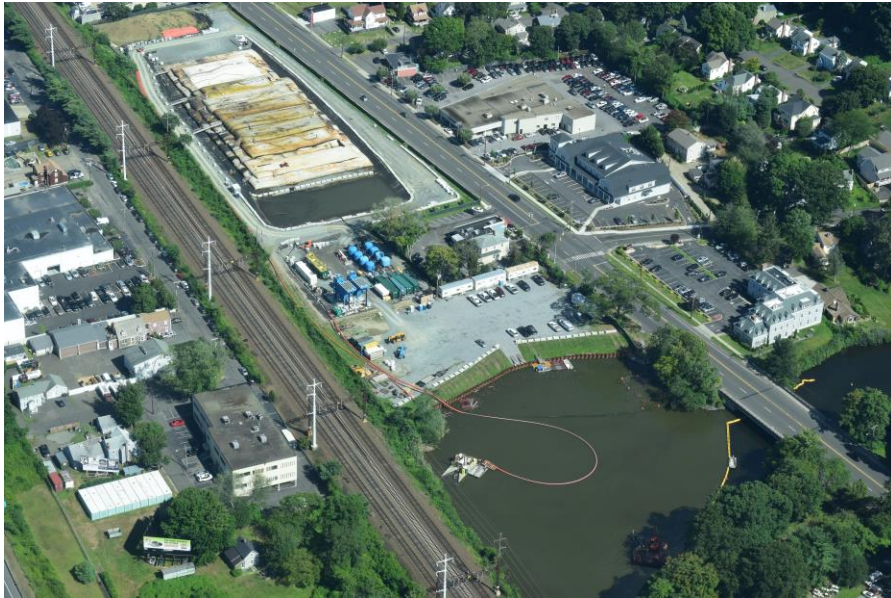
View during in-water remediation operations (8.13.2015)
