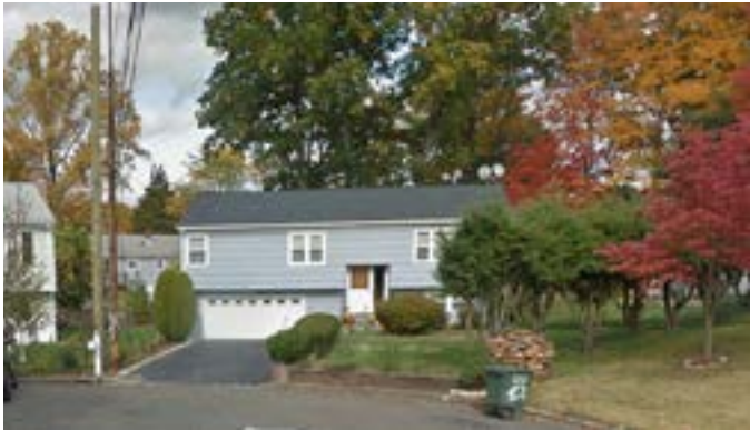
Figure 3.120-A. Examples of House D Building Type
