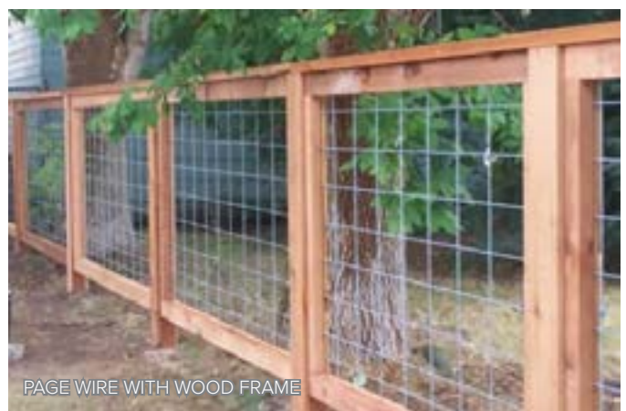
Figure 7-H. Examples of Fence Materials
