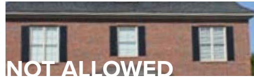
Inappropriately Sized Shutters.
