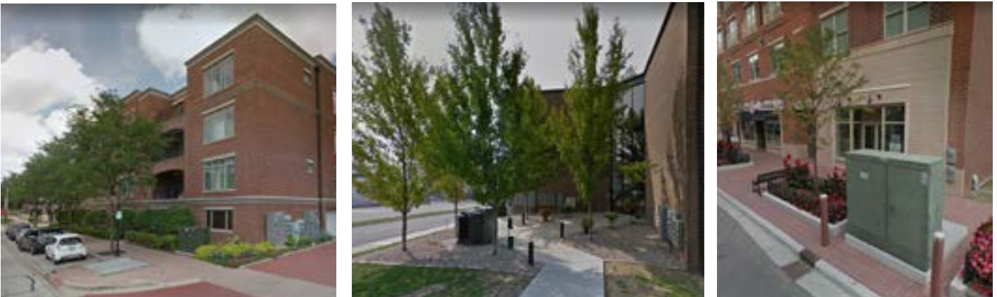
Figure 6-V. Examples of Poorly Located Utility Appurtenances on Primary Streets
