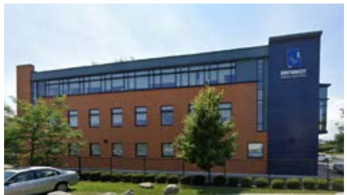
Figure 3.50-A. Examples of General Building Type
