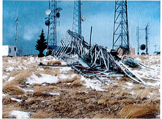
Cell tower collapses in high winds. Ruidoso, NM, Dec 18, 2009
