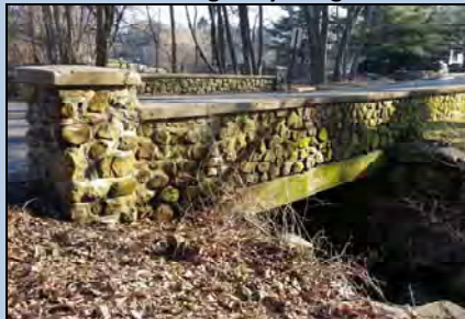
Cross Highway Bridge
