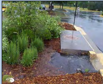
A Landscaped Island Used to Detain, Cleanse And Infiltrate Stormwater
