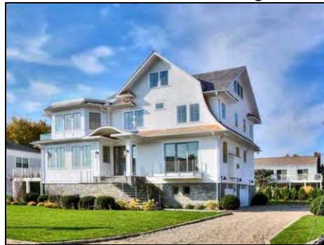
House Elevated To Flood Height
