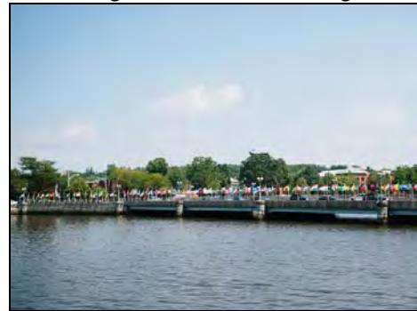
Rising Water At Post Road Bridge
