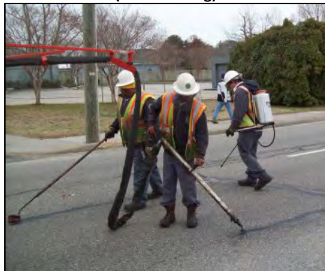
Pavement Management (Crack Sealing)
