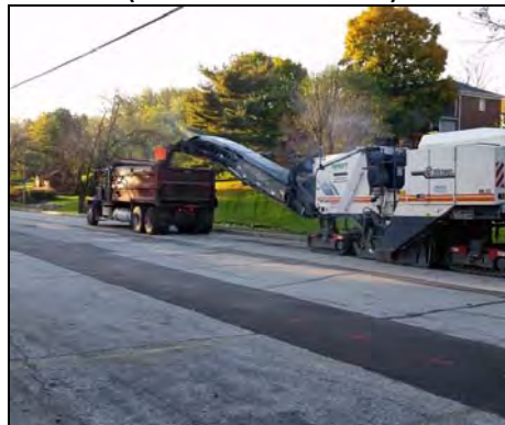
Pavement Management (Pavement Reclamation)
