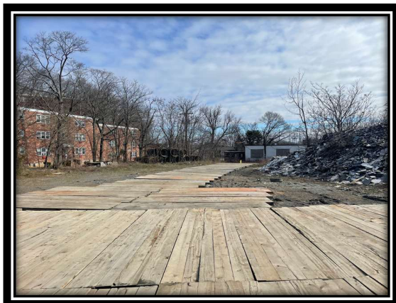
Photo 13: Temporary matted access road and work pad associated with P1026N. Accumulated stockpile associated with property owner's activities.
