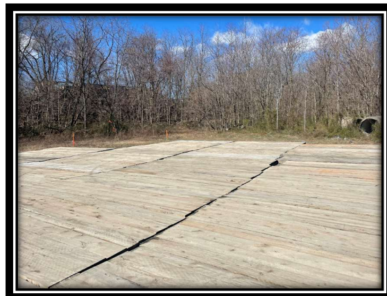
Photo 13: Temporary matted access road and work pad associated with P1026N. Accumulated stockpile associated with property owner's activities.
