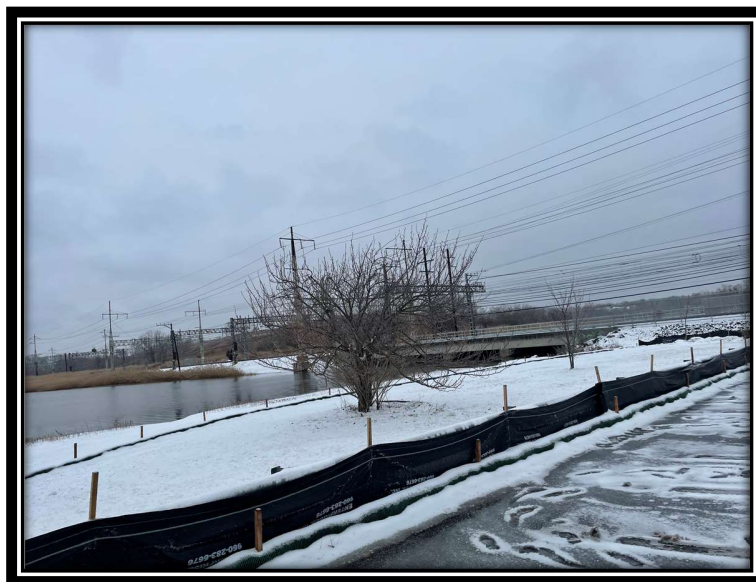
Photo 15: Exclusionary fencing associated with P1049S and P1049ES work pad.
