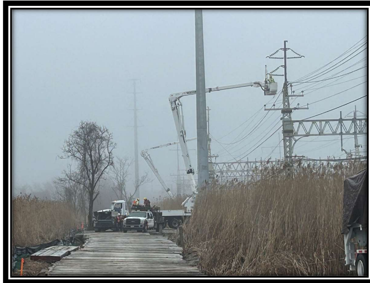
Photo 8: Typical bonnet removal.
