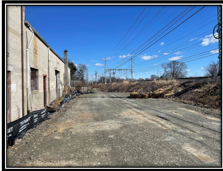
Photo 12: Temporary/permanent gravel access road to P1028N and P1027N.
