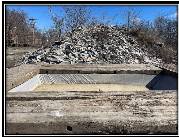
Photo 11: Concrete washout bin. Adjacent stockpile from property owner.
