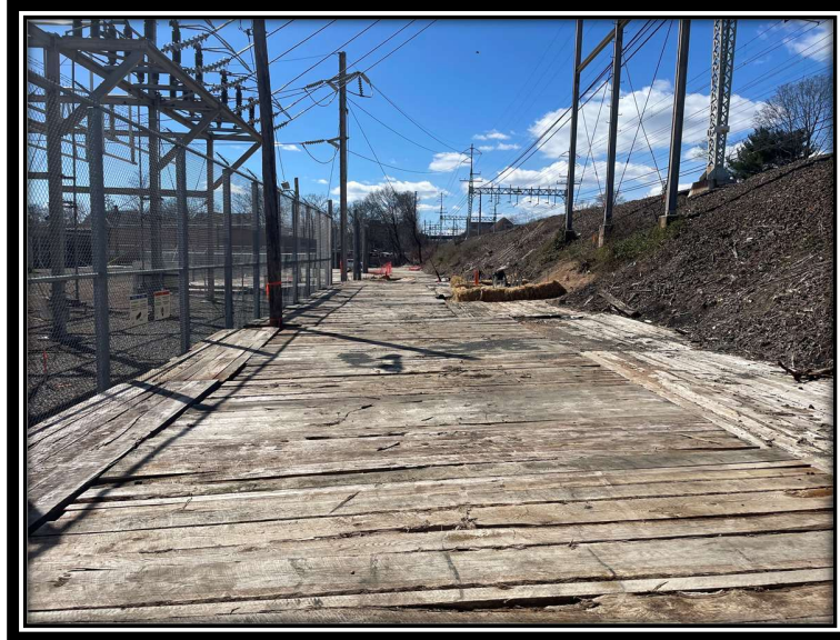
Photo 14: Work pad associated with P1029ES, P1029WNS, P1029SS, and P1028S, facing southwest.
