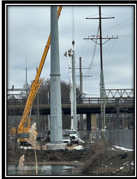
Photo 6: P1049N and P1049EN setting, located on east side of the West River.
