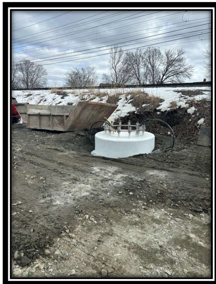
Photo 5: Typical cage setting for foundation concrete pour.
