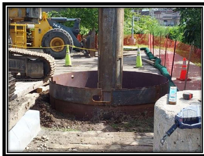
Photo 4 : Foundation drilling, typical.
