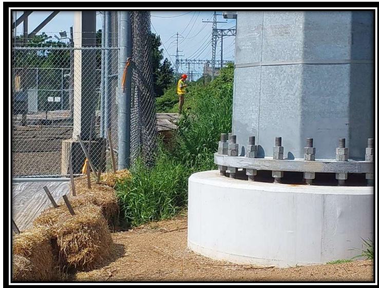
Photo 7: Constructed monopole base, typical.
