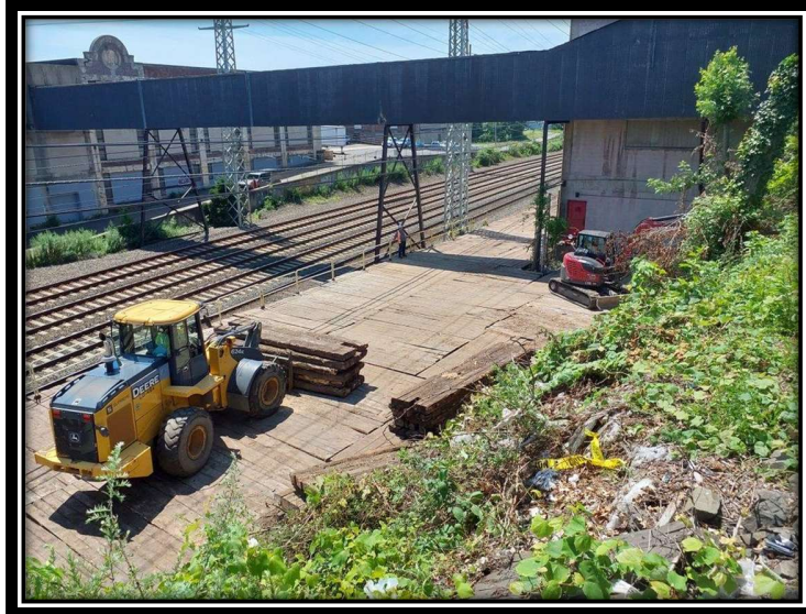
Photo 8: Matting placement activities, typical.
