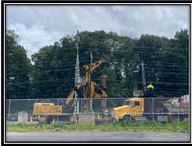
Photo 6: Foundation drilling, typical.
