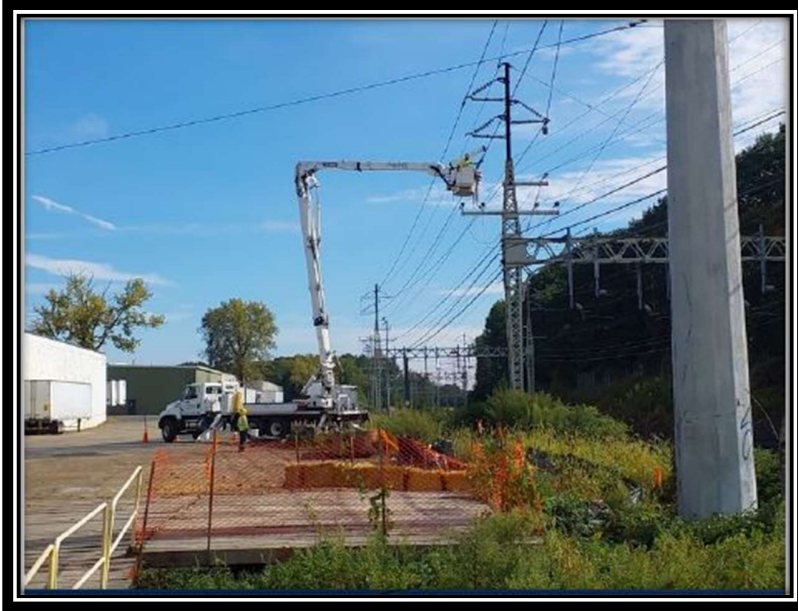
Photo 1: Typical bonnet removal.
