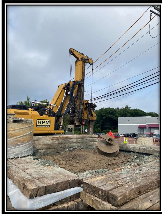
Photo 10: Spinoff bin for drilling activities, lined with impermeable polyethylene sheeting, typical.
