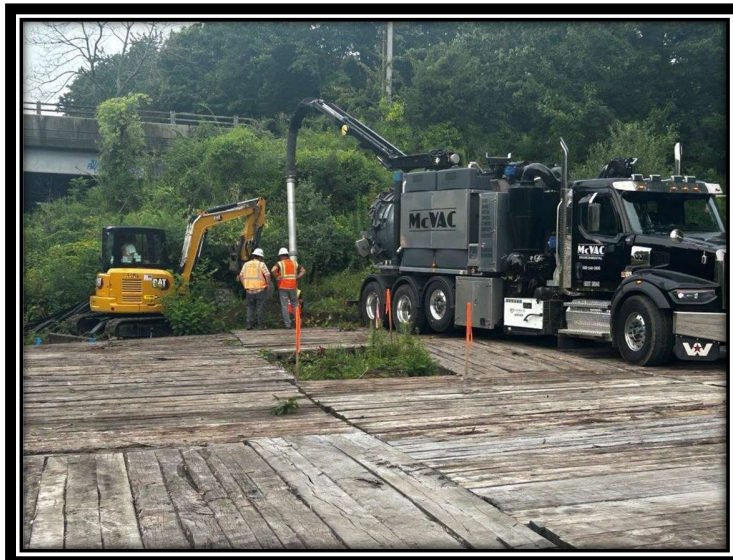
Photo 9: Soft dig activities, typical.
