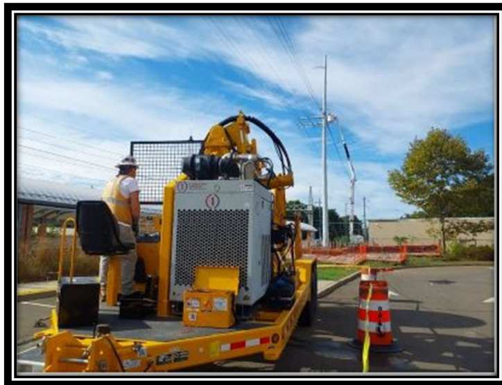
Photo 6: Conductor pull, typical.
