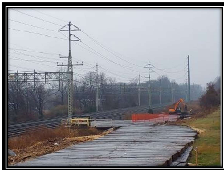
Photo 6: Matting placement activities, typical.
