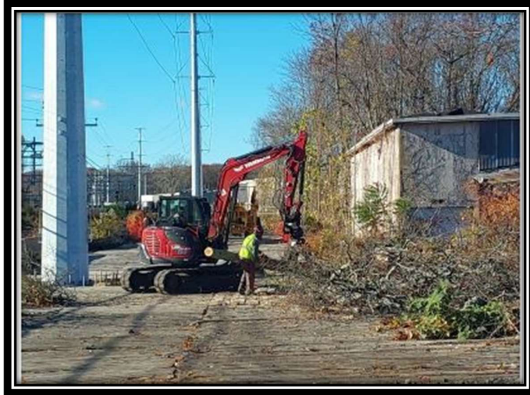
Photo 7: Vegetation removal, typical.
