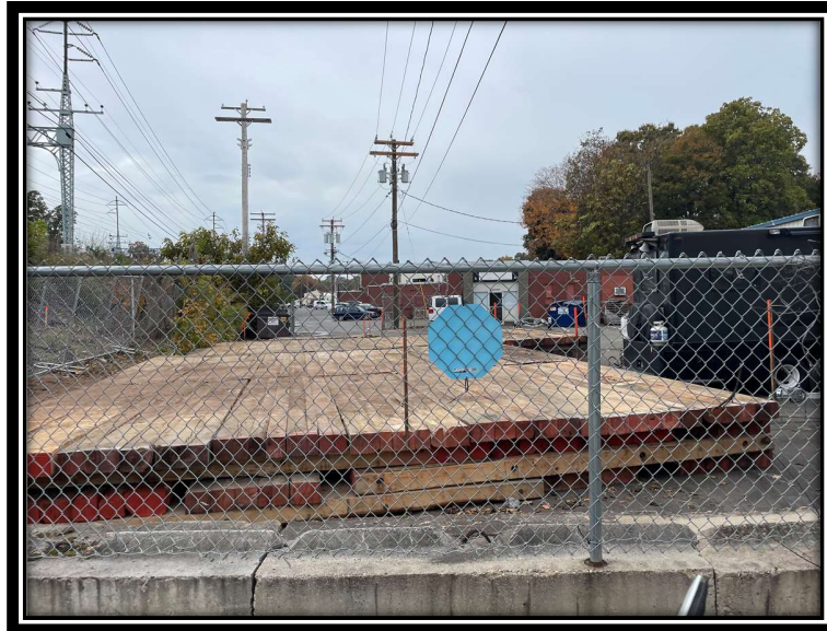
Photo 11: Work pad associated with P1033N, facing west and towards York Street.
