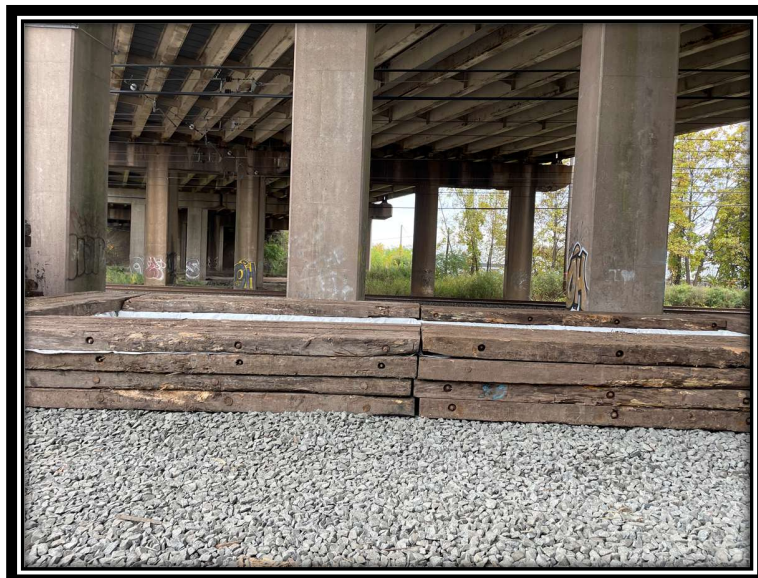
Photo 8: Concrete washout, located off Mix Avenue.
