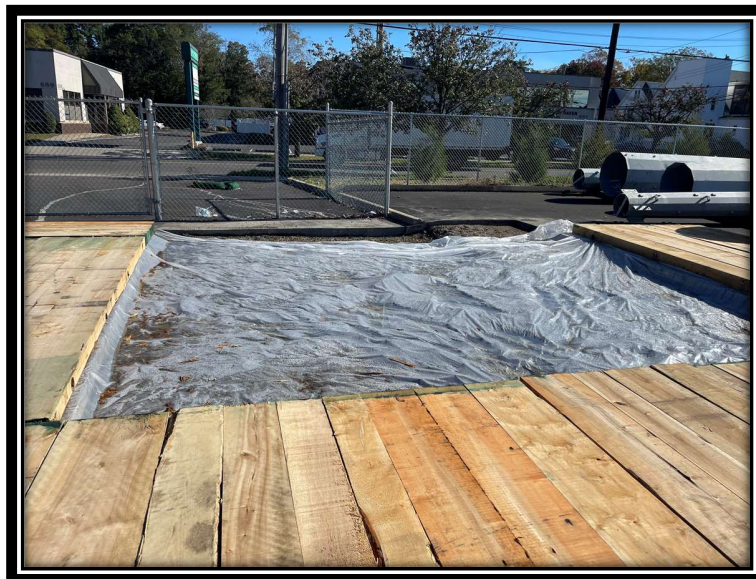
Photo 4: Covered soft-dig location at P1030S, with surrounding work pad matting.
