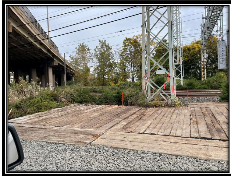
Photo 19: Work pad associated with P1041N.
