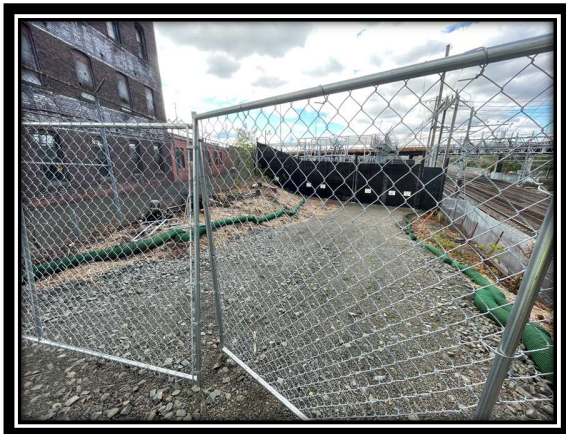
Photo 2: Permanent road installation off Grant Street and into the West River Substation. Completed with erosion controls, mulching, and seeding.
