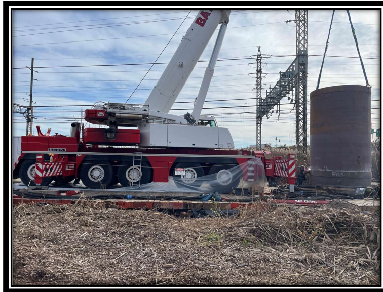
Photo 13: Caisson installation at P1043N.
