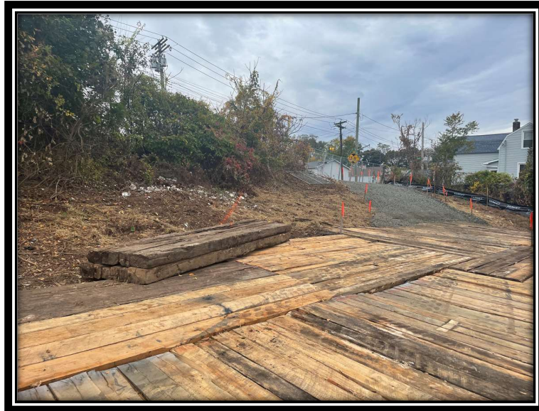
Photo 7: Work and tracking pad installation associated with P1039N.
