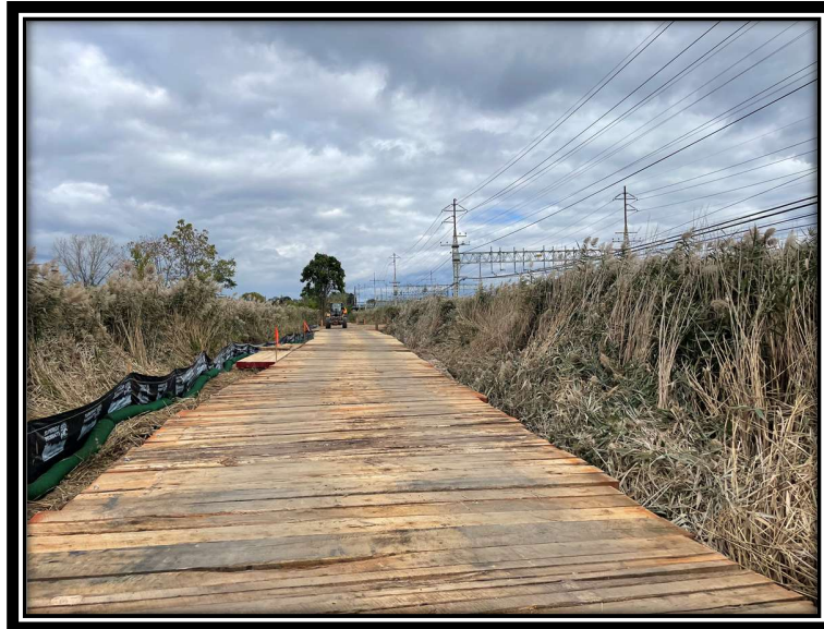
Photo 3: Matting through wetland area, located on western side of the West River, facing east.
