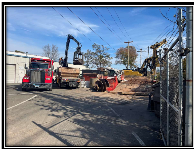
Photo 12: Active drilling activity with soil spin-off associated with P1033N, facing east.
