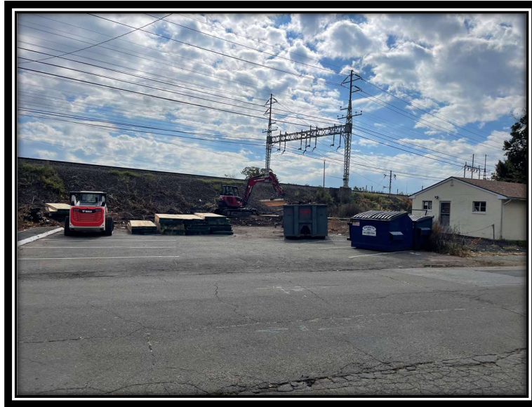
Photo 5: Vegetation clearing and work pad installation associated with P1030N.
