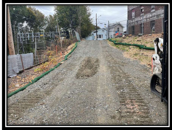
Photo 2: Permanent road installation off Grant Street and into the West River Substation. Completed with erosion controls, mulching, and seeding.
