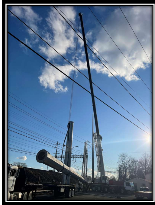
Photo 15: Structure installation at P1030N.
