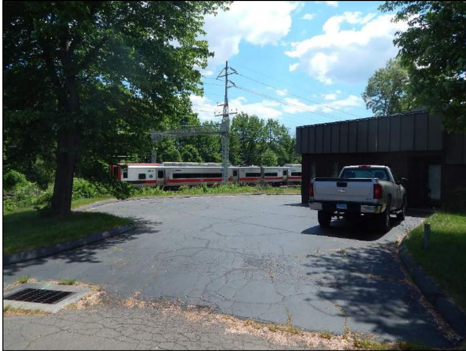
Figure 24. Overview photo taken from Higgins Drive in Milford toward proposed access road and work/pulling pad.
