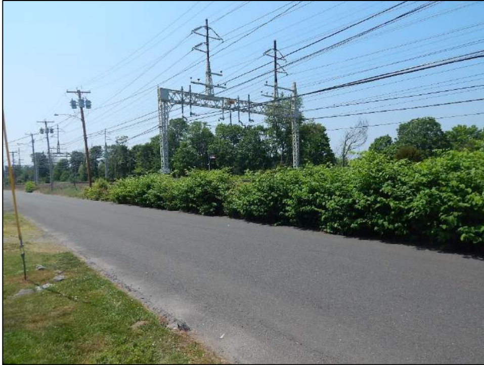
Figure 28. Overview photo taken from Buckingham Avenue looking west toward proposed work/pulling pad along the existing CT DOT corridor in Milford.
