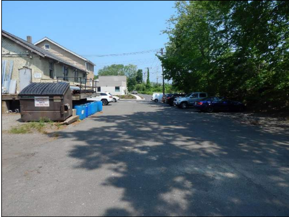
Figure 20. Overview photo looking East showing proposed access road connecting proposed work pull pad to Gulf Street in Milford.
