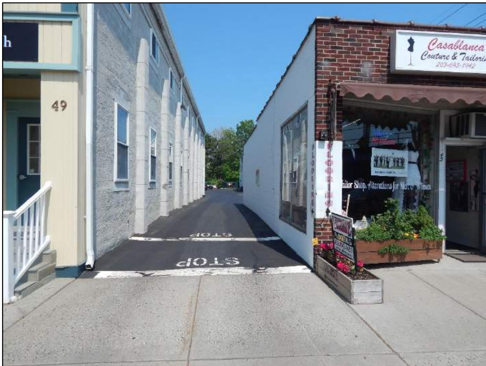
Figure 21. Overview photo taken from River Street looking east along proposed access road in Milford.
