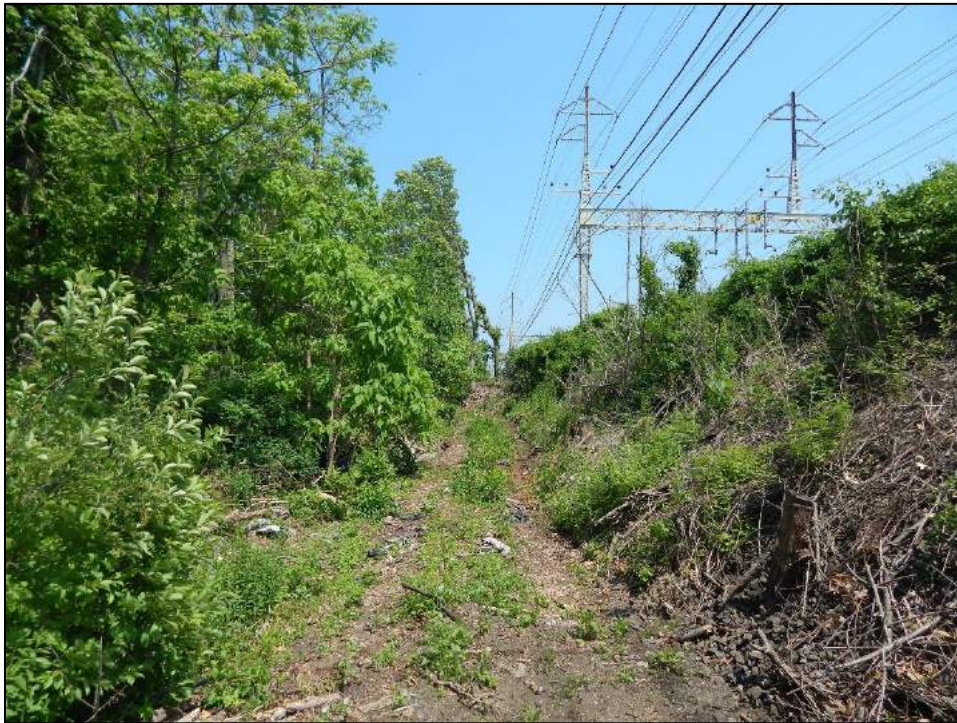
Figure 18. Overview photo of proposed work/pulling pad looking east along the existing CT DOT corridor toward Gulf Street in Milford.
