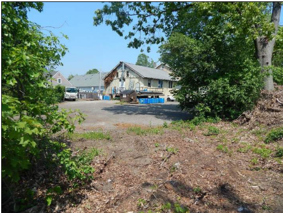
Figure 19. Overview photo taken from proposed work/pulling pad looking northeast toward proposed access road connecting to Gulf Street in Milford.
