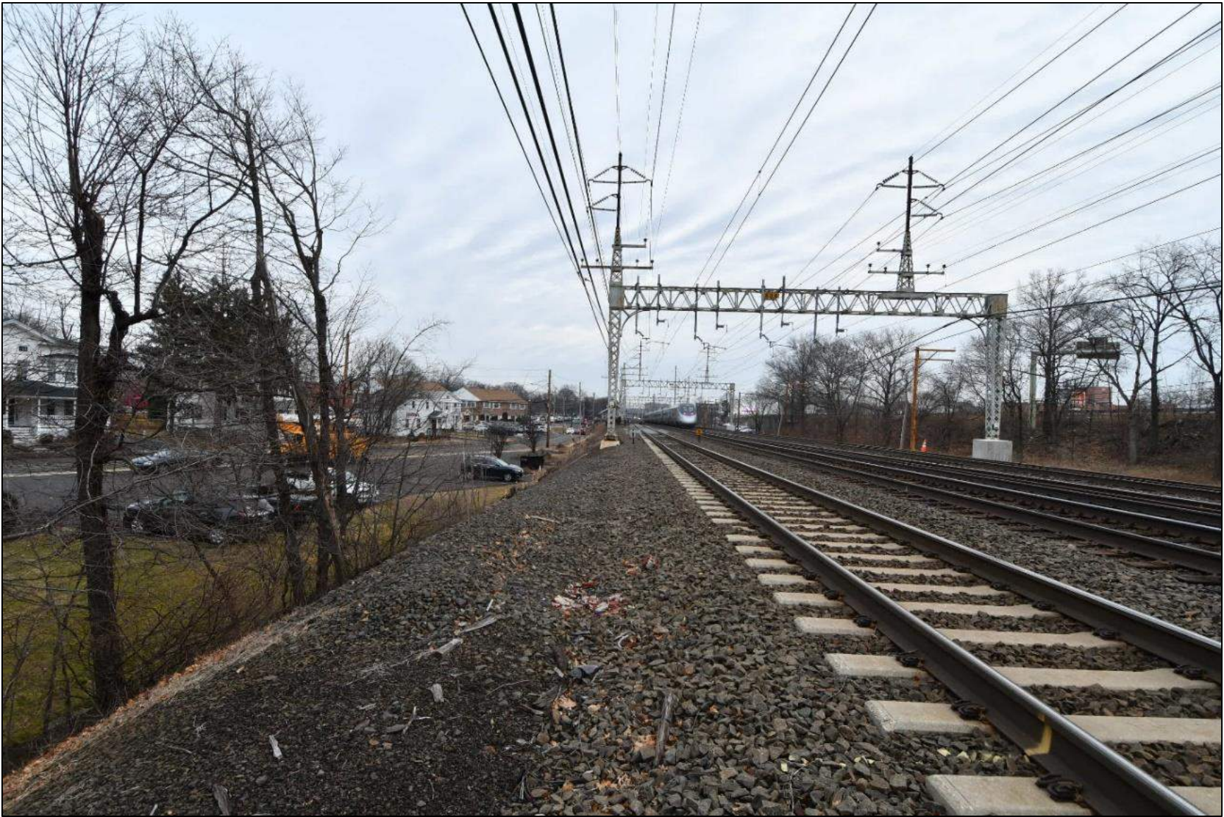
Figure 14. Overview photo of pre-construction conditions along an adjacent section of the existing CT DOT corridor.
