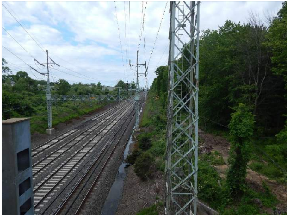
Figure 33. Overview photo taken from the Allings Crossing Road bridge crossing in West Haven. The view is southwest.
