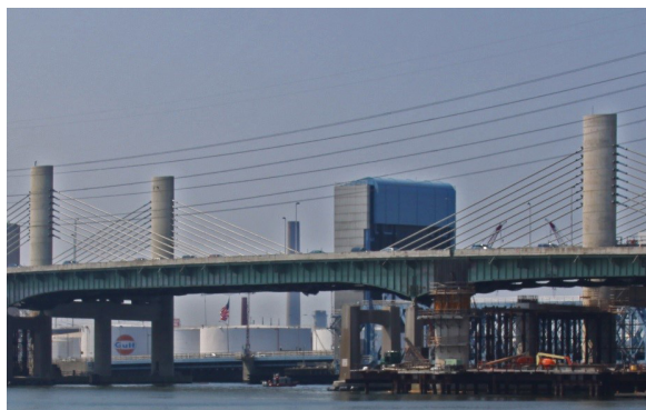
View of the partially constructed Q bridge in New Haven overlooking Quinnipiac river. More than 150,000 vehicles cross this bridge per day (2006 ConnDOT data).
