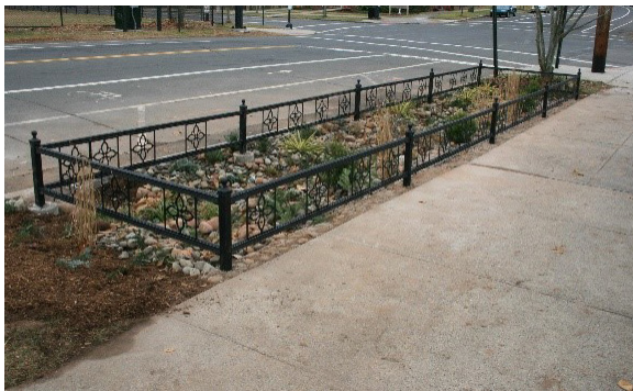
View of recently installed bioswale at Edgewood School. With the help of federal grant money, the City plans on installing nearly 200 bioswales all across the city, within the next two to three years, to manage stormwater runoff effectively.
