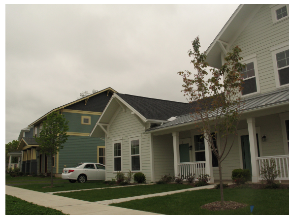
Recently re-built government-assisted Brookside housing development in West Rock neighborhood.
