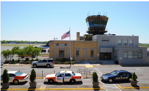
Tweed New Haven Airport's passenger terminal and parking area have the operational capacity to accommodate a substantial increase in scheduled airline service. Economic and runway length issues have so far hampered efforts to attract additional air carriers.
