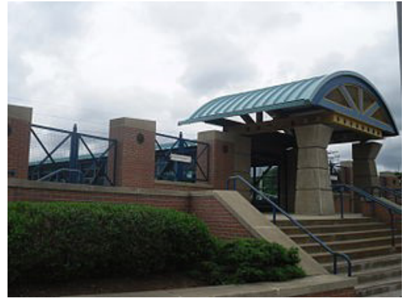
View of State Street Train Station
