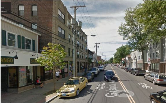
Transforming Grand Avenue into a Main Street is one of the priorities for Fair Haven neighborhood for the next decade.
