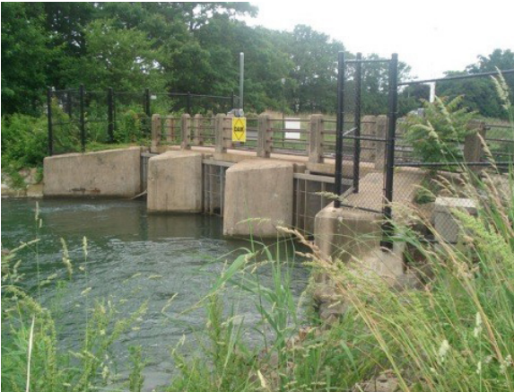
Floodgates installed at Dean Street in Morris Cove neighborhood.
