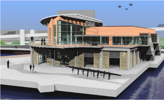
Rendering of the Boathouse facility at Canal Dock currently under construction which will reconnect city residents with the waterfront and provide a focal point for community-oriented recreational/educational programs.
