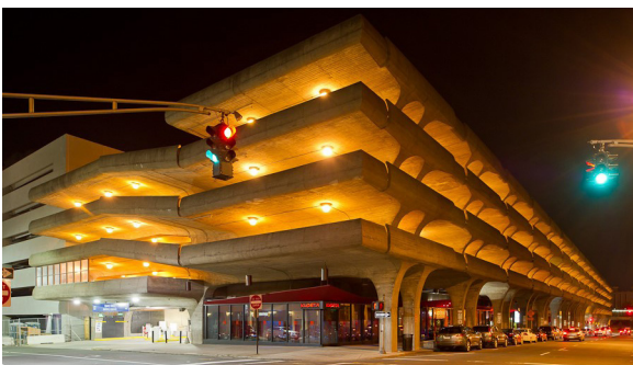
The creation of ground floor retail spaces as “liners” for parking structures, such as the Temple Street Garage (above), allows the continuation of the pedestrian-oriented street frontage.
