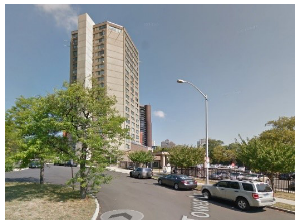
Example of a high-density residential property located on Tower Lane
