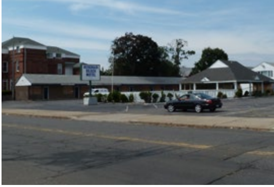
The vacant Debonair motel on Beach Street
