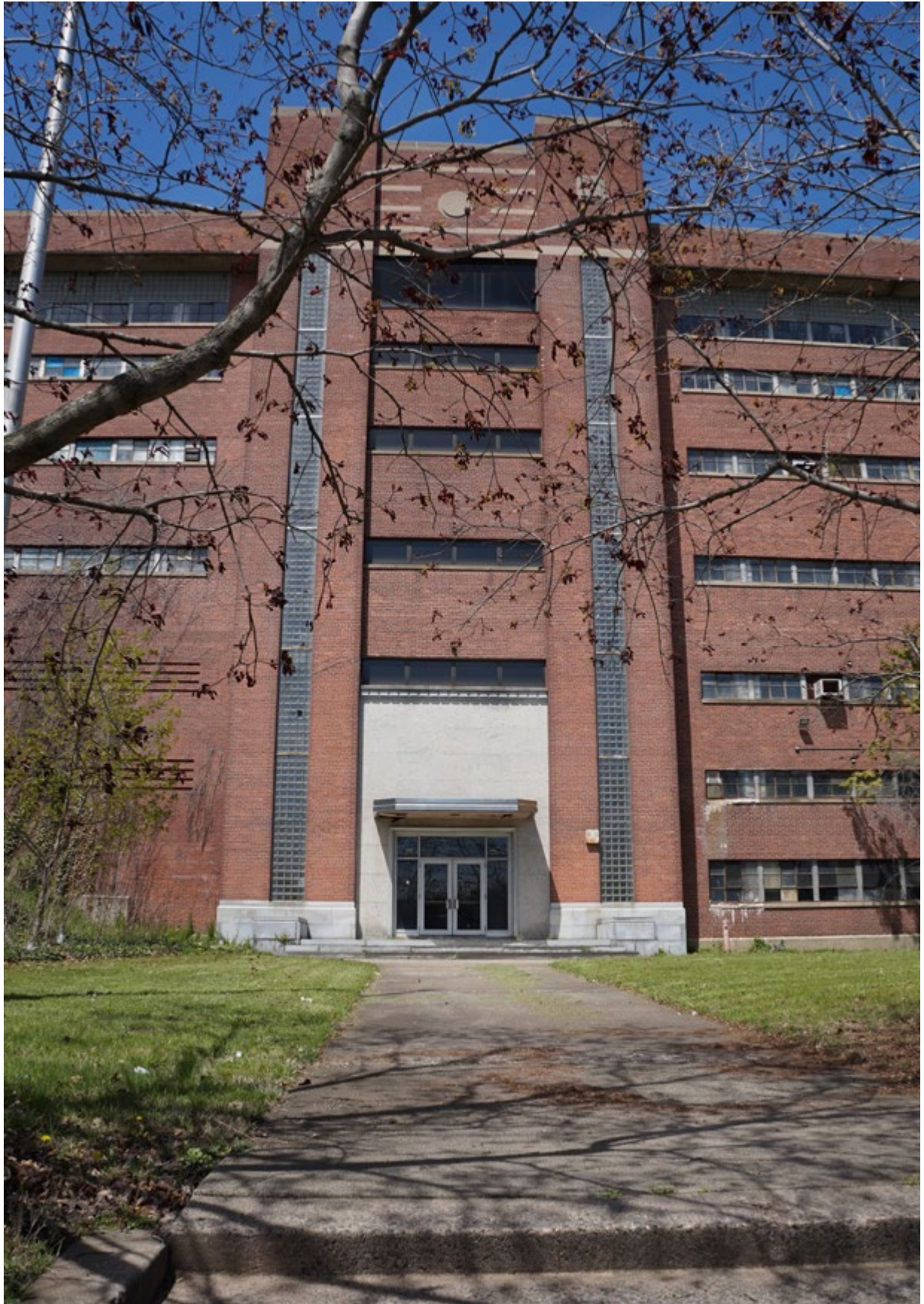
The former Armstrong Tire Company building on Elm Street
