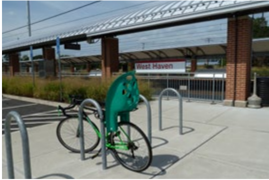
West Haven Station
