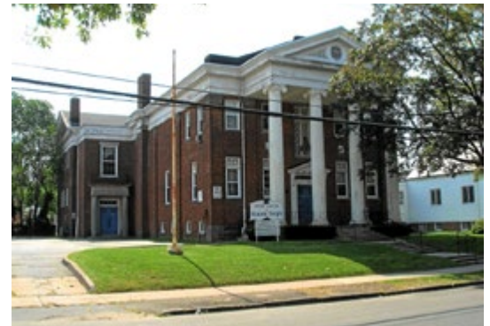
P-D7. The former Masonic Temple will be converted into the West Haven Center for the Arts.
