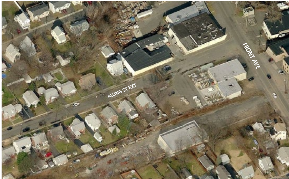
P-A3. In the Front Avenue corridor, commercial and industrial buildings are located in close proximity to residential homes—in some instances without any protective buffer.
