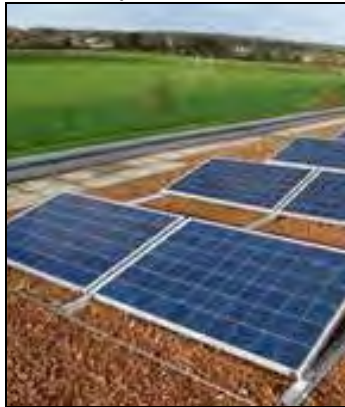
Rooftop Solar Installation
