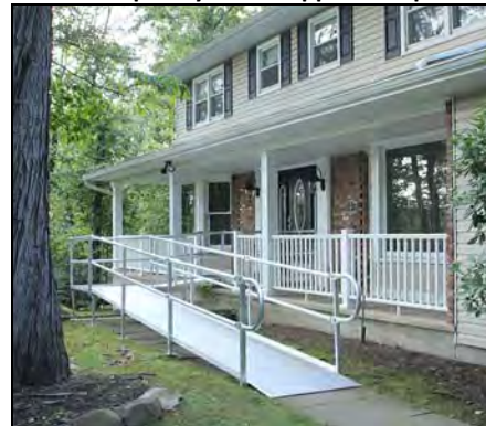
Temporary Handicapped Ramp
