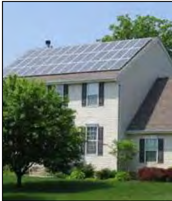
Residential Solar Installation
