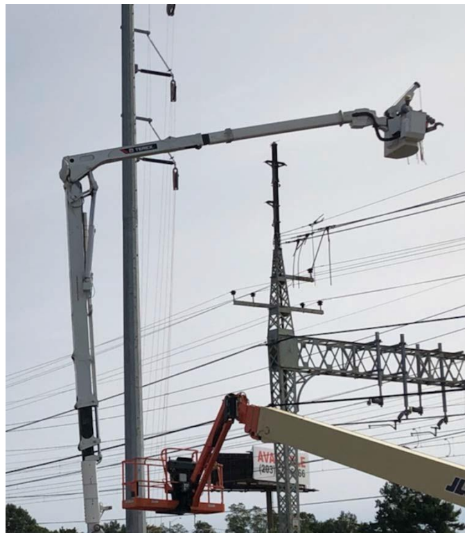
Figure 2-3: Wires Temporarily Tied Off on One Side at Base of Bonnet
