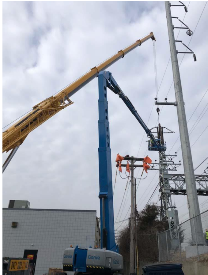
Figure 2-4: Bonnet Removal from Catenary Structure
