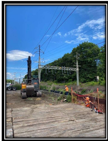
Photo 6: Safety and E&S controls installation-typical.
