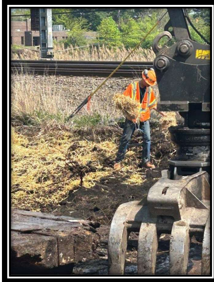
Photo 12: West River wetland restoration process-straw cover prior to revegetation.
