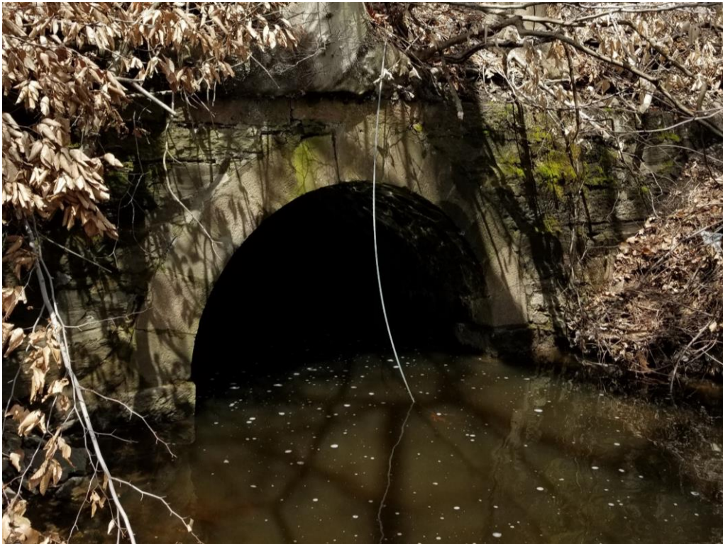
PHOTO 9: Downstream view of Cove River, looking north at the culvert outfall.
