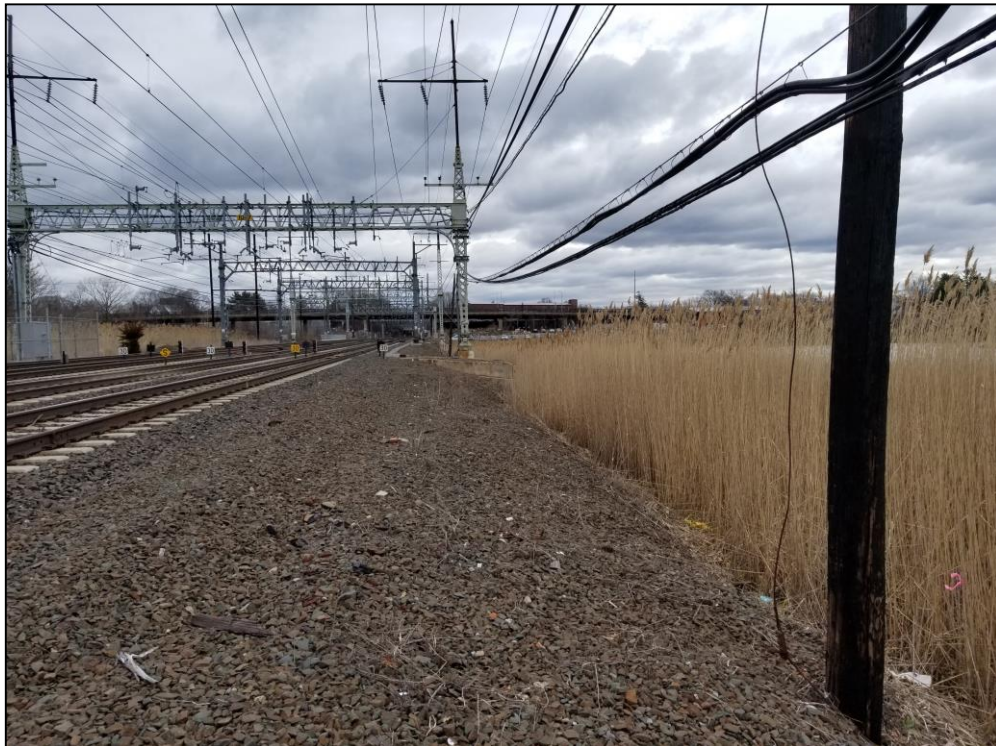
PHOTO 2: View of Wetland 1, looking east from the tracks towards West River.
