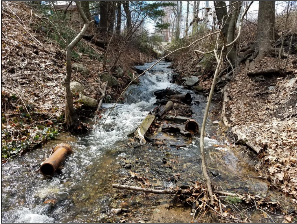
PHOTO 7: View of Stream 1, looking west from the toe of slope.
