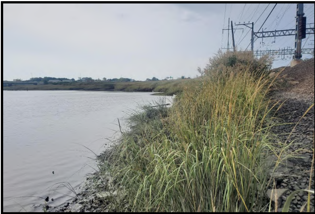
Photo 10: Southern portion of West River survey area. Photo taken looking west. 9/28/2021.
