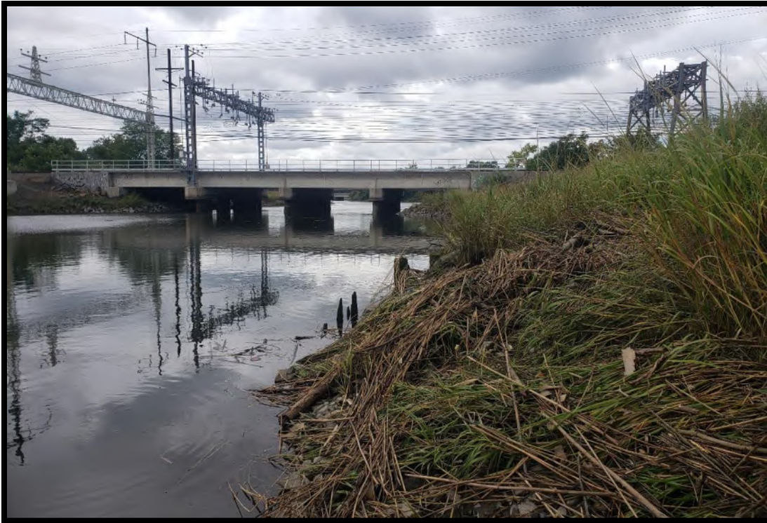
Photo 11: Eastern portion of West River survey area. Photo taken looking north. 9/16/2021
