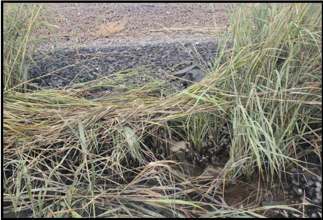
Photo 73: Rip-rap slope of MNR corridor, with a thin bank of native vegetation, comprised of smooth cordgrass. Photo taken looking northwest. 9/28/2021.
