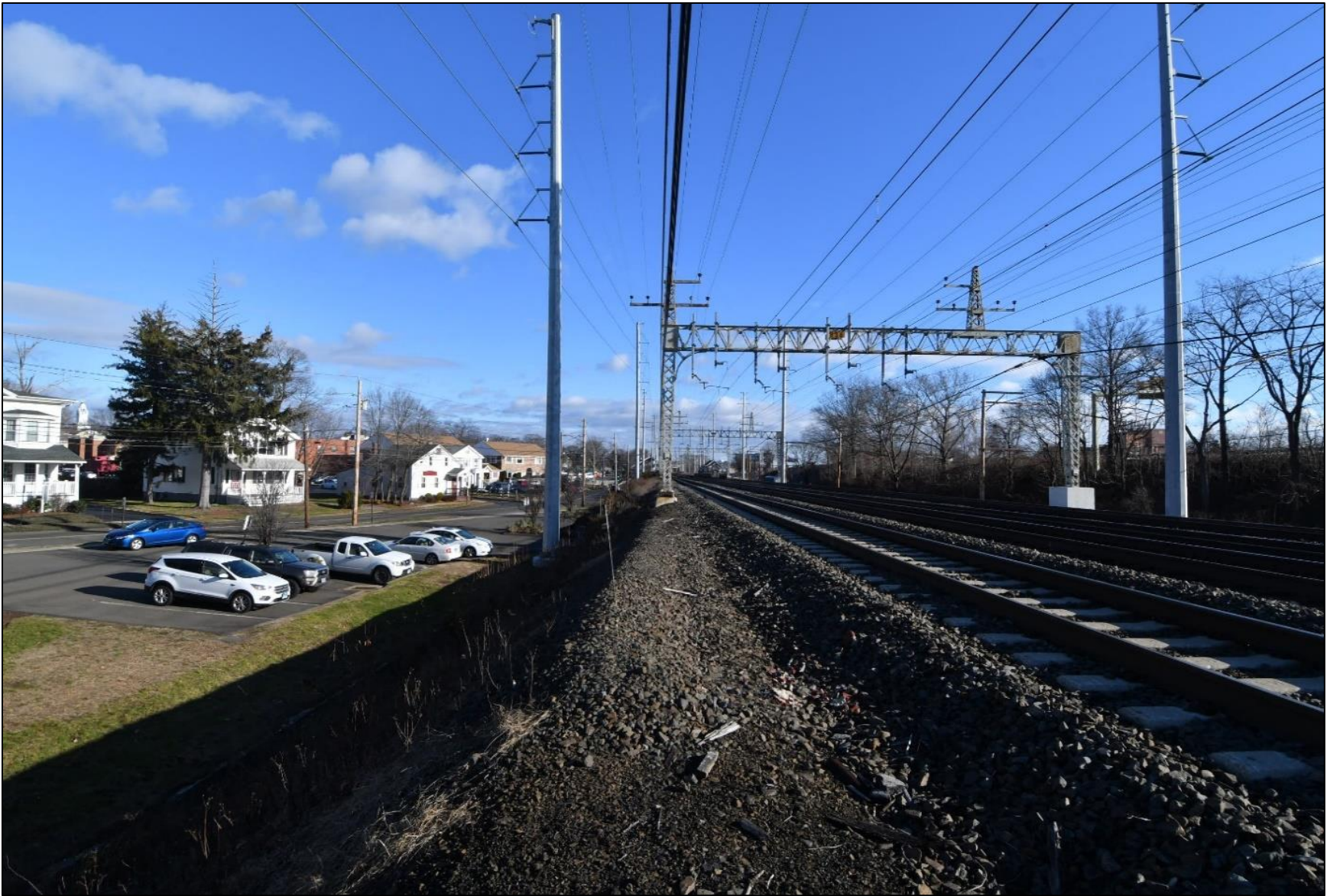
Figure 5. Overview photo of post-construction conditions at HRX-Baird Pole 838N.
