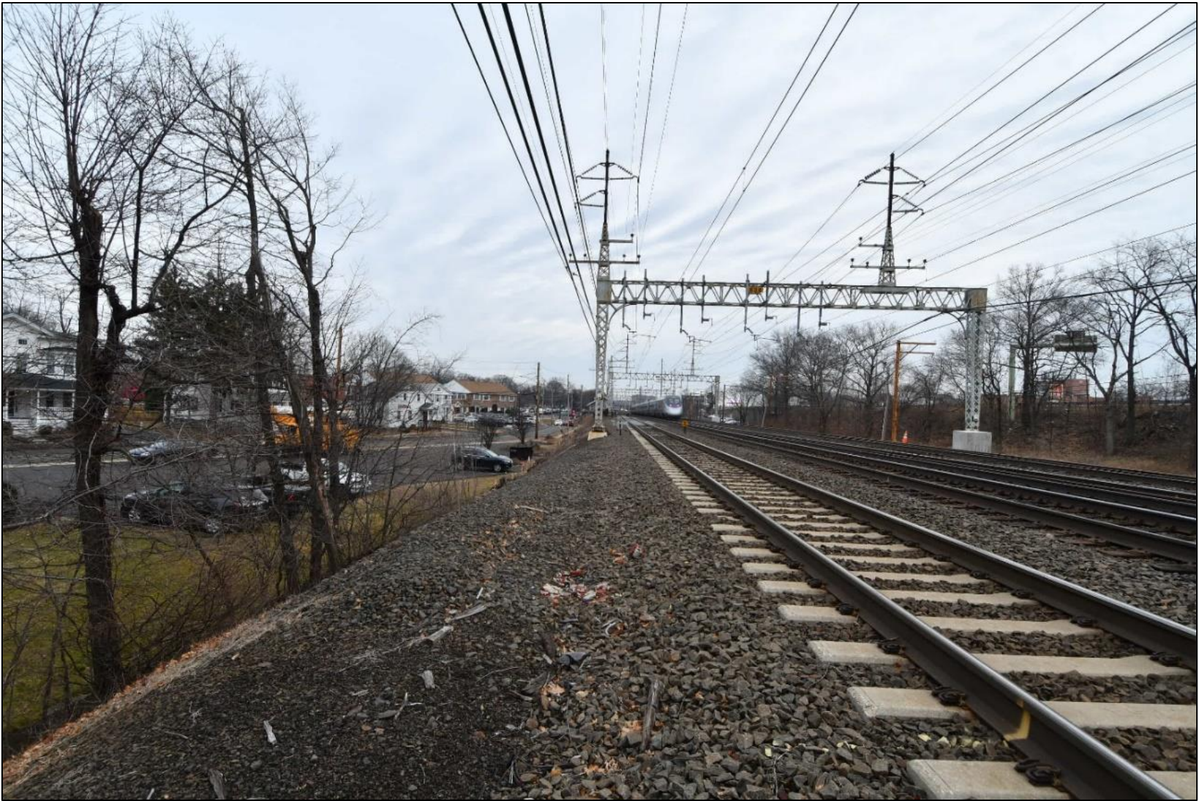
Figure 4. Overview photo of pre-construction conditions at HRX-Baird Pole 838N.
