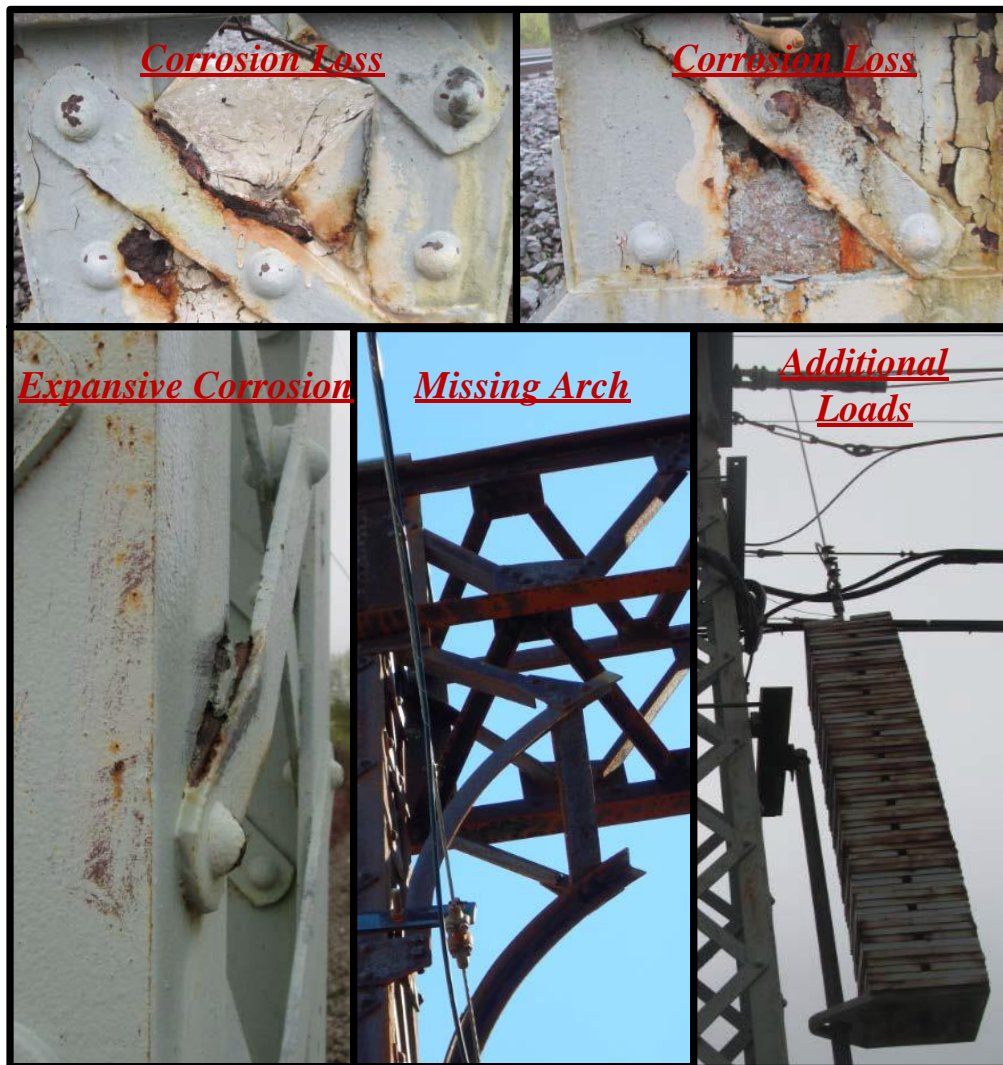
Figure 3.1: Field Condition Visuals
