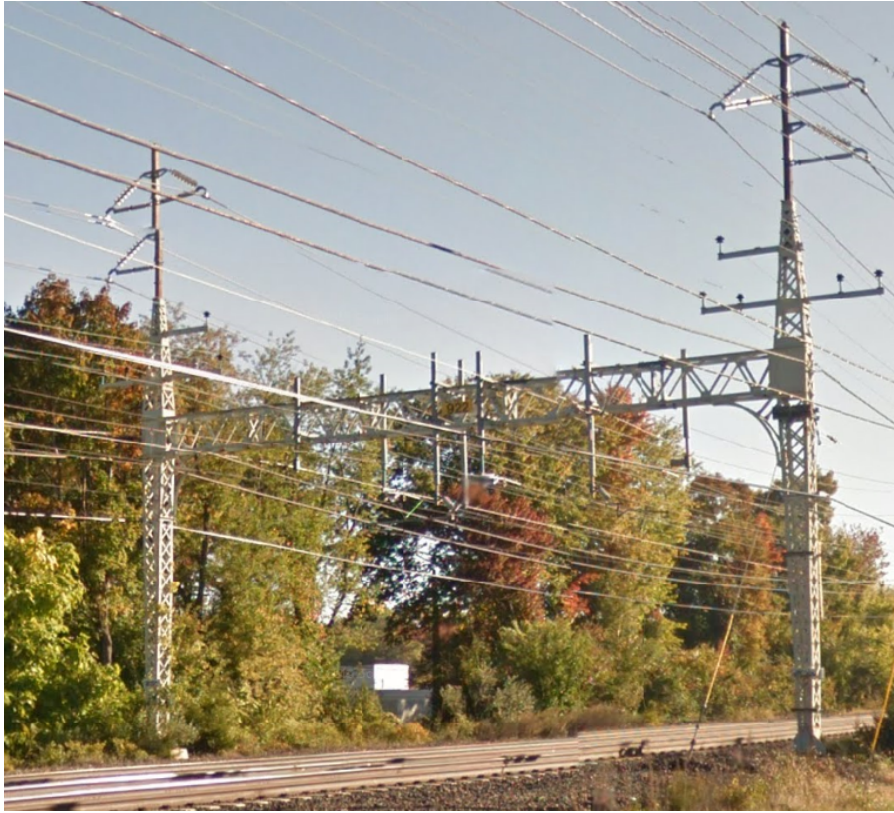
Figure 3: Typical Existing structure (Structure Type 1&2 - #922 Shown)
