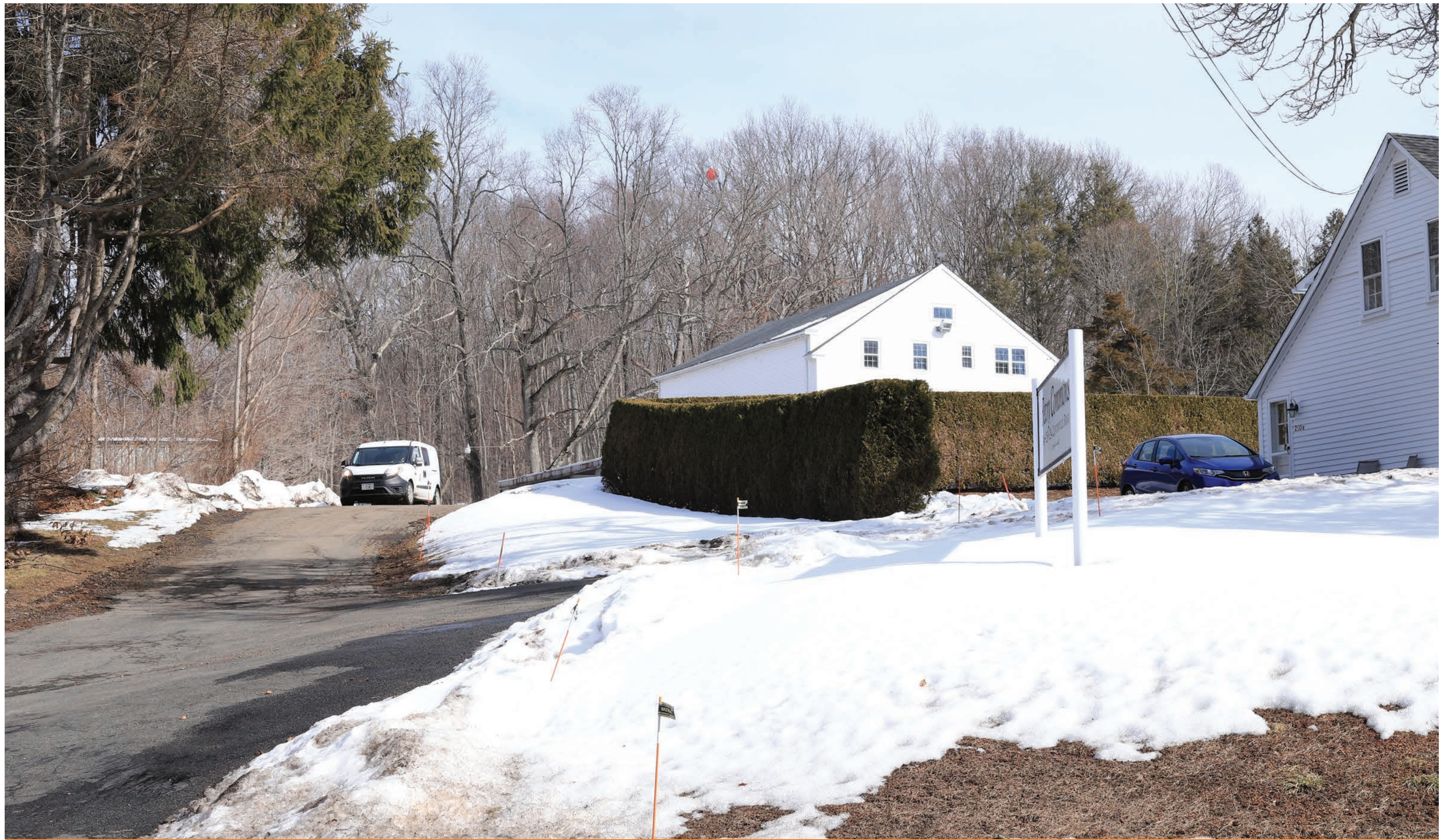
Photo 65 - Clintonville Road near #250 EXISTING CONDITION
