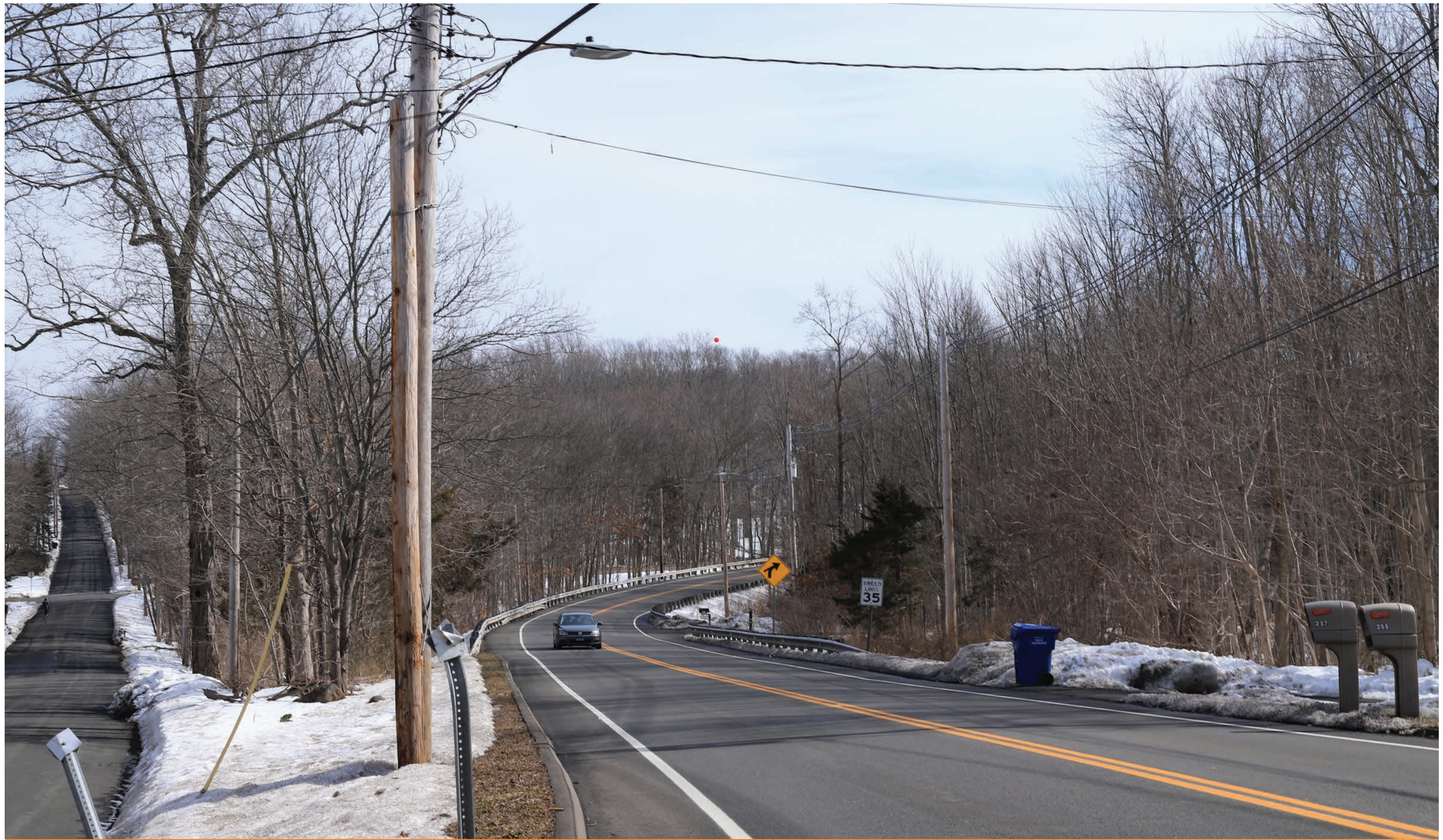
Photo 68 - Clintonville Road near Pistapaug Road EXISTING CONDITION
