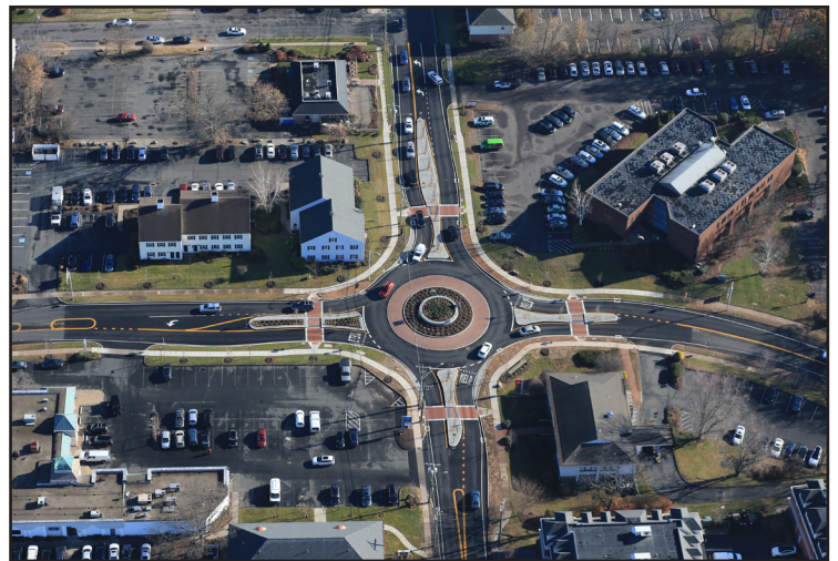
Traffic roundabout at Hebron Avenue and New London Turnpike
