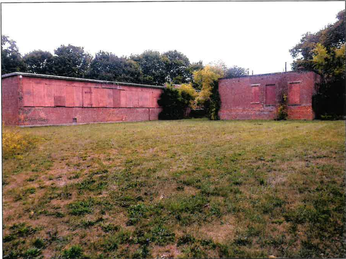
Photo 6. Overview photo showing proposed monopole location in New Britain, Connecticut. View is southeast toward former Israel Putnam Elementary School in New Britain, Connecticut.
