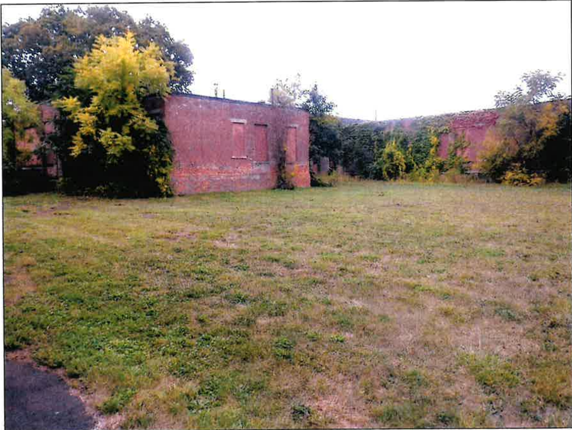
Photo 7. Overview photo showing proposed monopole location in New Britain, Connecticut. View is southwest toward former Israel Putnam Elementary School in New Britain, Connecticut.
