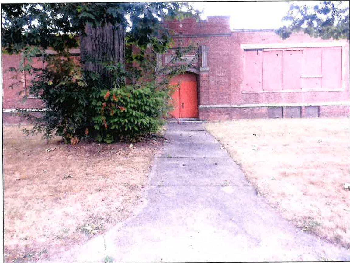
Photo 11. Overview photo taken from Osgood Avenue showing main entrance to the former Israel Putnam Elementary School in New Britain, Connecticut.
