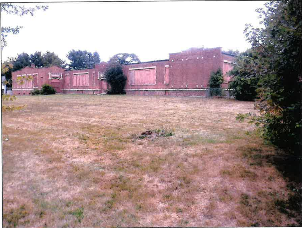
Photo 10. Overview photo taken from the intersection of Osgood Avenue and Beach Street looking northeast toward southwest corner of former Israel Putnam Elementary School in New Britain, Connecticut.
