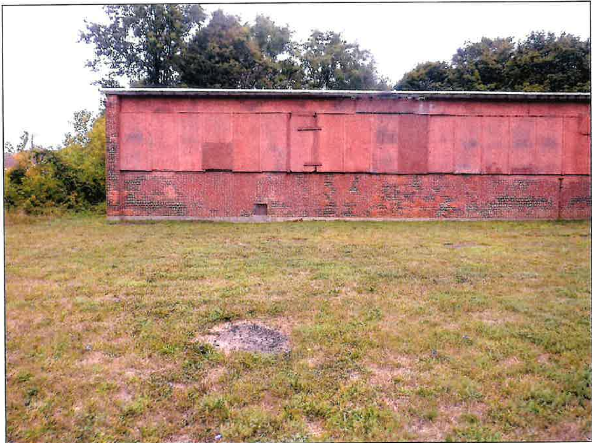
Photo 4. Overview photo from proposed monopole location looking east toward former Israel Putnam Elementary School in New Britain, Connecticut.
