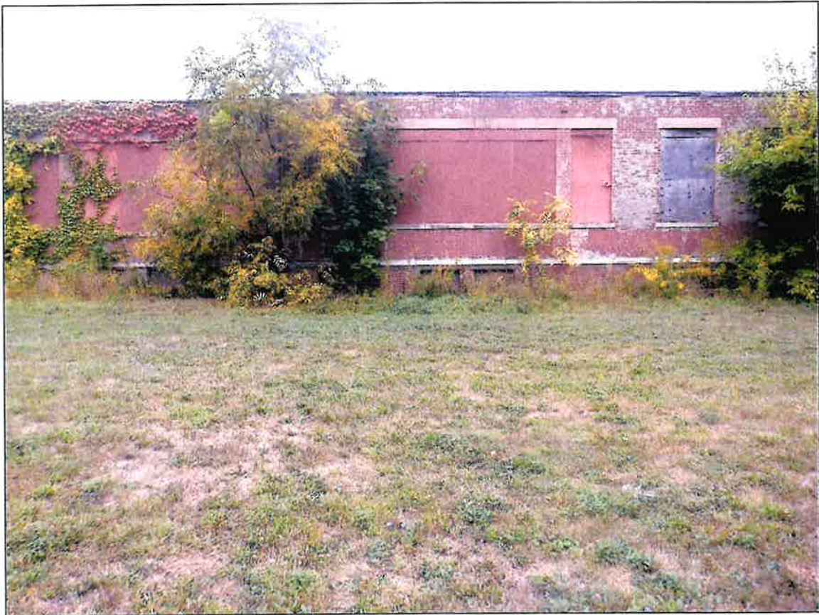
Photo 2. Overview photo from proposed monopole location looking west toward former Israel Putnam Elementary School in New Britain, Connecticut.
